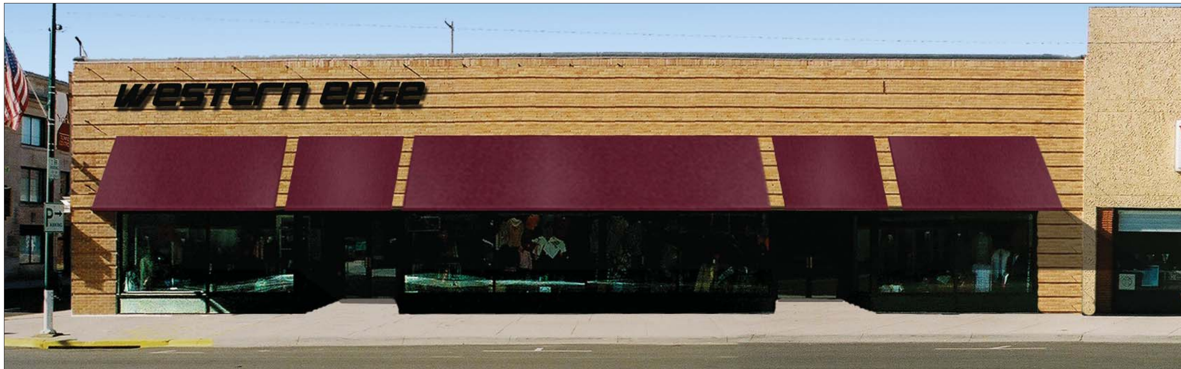
Image 4. Option 1. Awnings fabricated with Sunbrella's Burgundy (#4631) fabric articulate the store entrances and provide shading for the display windows, as well as weather protection for pedestrians. The signage, in "Bauer" font, is mounted to align with the awning at the corner of the building.
