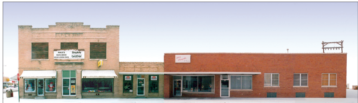
Image 1 (left). Existing condition of East Facade.
