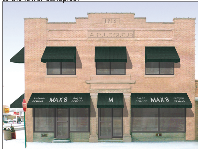
Image 6. Option 2 (east). The windows and window frames have been updated as in Option 1. Awnings in Sunbrella "Marine Blue" (#4678) to all windows and doors. Store signs are applied in white to the lower canopies.
