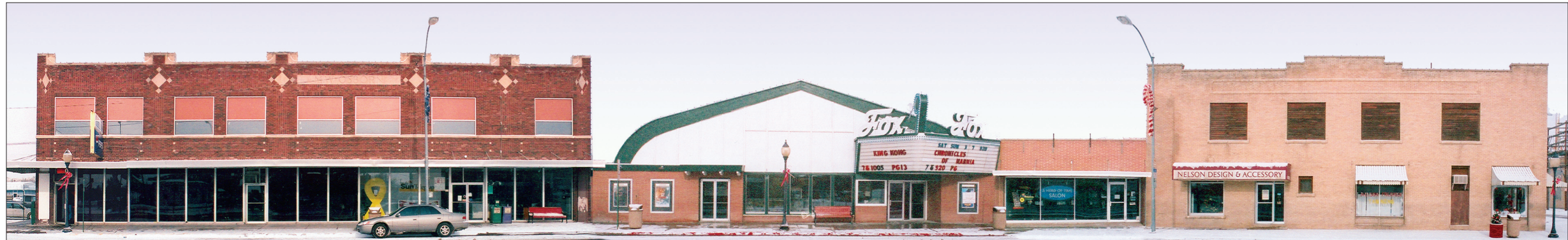
Image 2 (below). Existing condition of South Facade.
