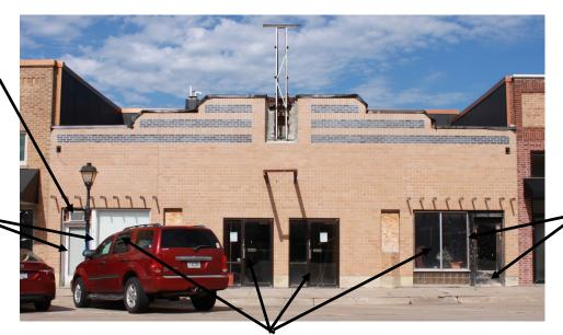
Repair deteriorated wood trim around the door/door frame and door. Paint a dark color to blend in with the center doors and other building trim.
