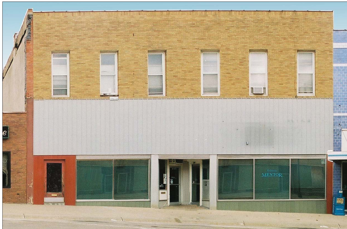
Image 2. Existing Condition. The Davidson Insurance & Real Estate office occupies the western (to the left in this image) half of the first floor of the two-story building at 808-810 Central Avenue. Apartments occupy the second story of the building. The first floor is divided equally into two tenant spaces, with recessed, angled entrance doors located at the party wall halfway across the building's full-width glass storefront. The large full-width signboard, extending from the top edge of the storefront to the bottom edges of the second story window sills, is sheathed with vertical metal siding.
