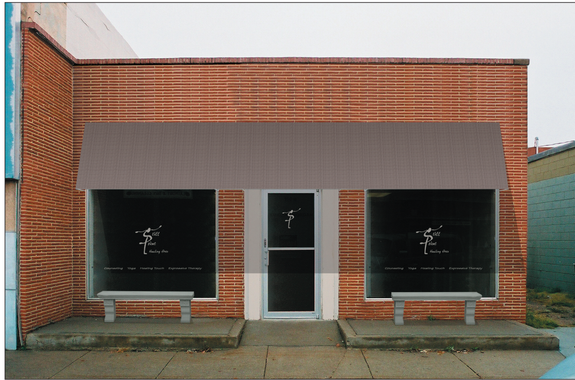
Image 9: Option 7. One continuous awning in Sunbrella fabric Linen Tweed (4654) is centered above the front windows and door. The awning is composed of a single plane; it has no sides or valance. The Still Point logo is applied to the two windows and to the top of the door glass. Two concrete benches are on either the concrete platforms that flank the door.
