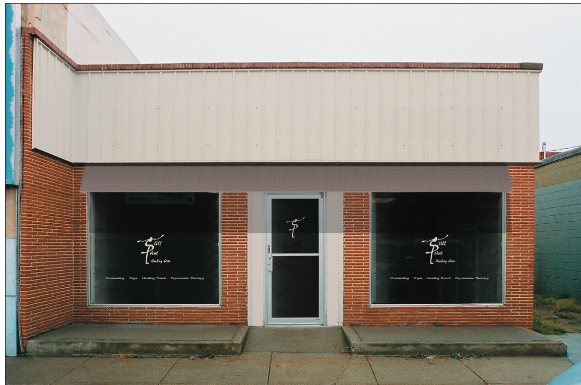
Image 3: Option 2. The awning composition is the same as in Option 1 and is in Sunbrella fabric Linen Tweed (4654). The metal siding and door frame are painted off-white, and the window logos are in a similar color.
