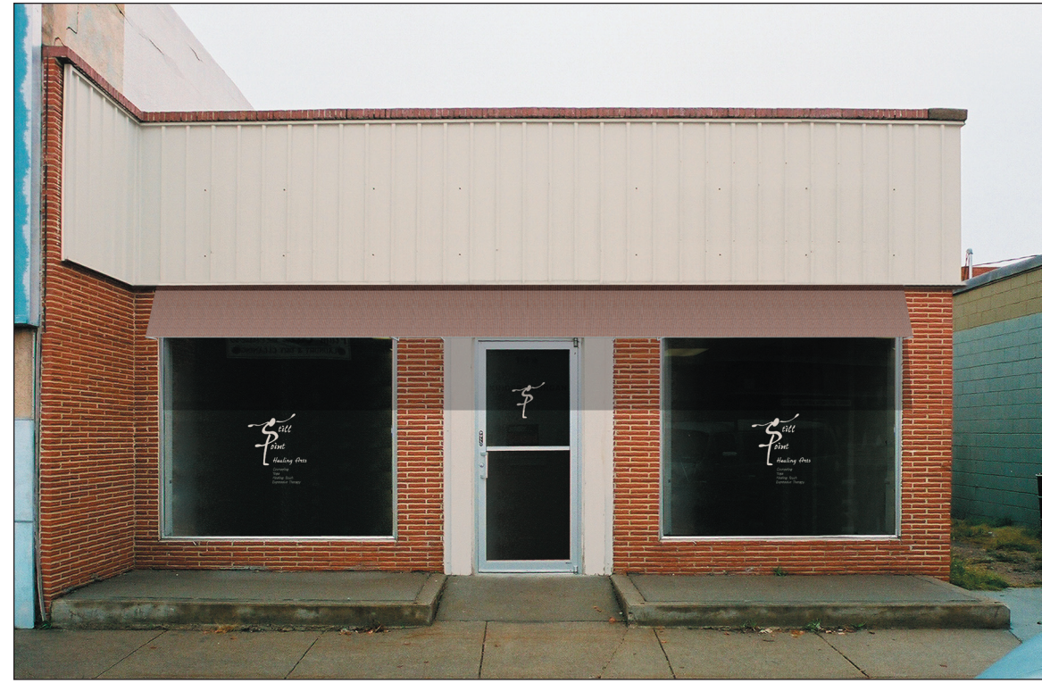
Image 2: Option 1. One continuous, "eyebrow" awning in Sunbrella fabric Mocha (4616) is centered above the two windows and door. The awning is composed of a single angled plane and is placed just below the metal siding. Its bottom edge ends just above the top of the front door. The door frame and the metal siding are painted an off-white color. Logos have been applied to the windows in the same off-white color. The full-height glass in the front door is restored.
