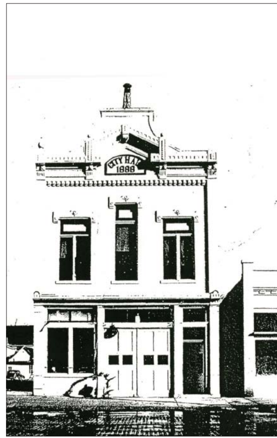
Image 2. Historic Photograph. In later years the building was used as a fire hall. A large garage door to accommodate fire fighting equipment was added, thereby significantly altering the first story front façade of the building. The original second story had an unusually high floor-to-ceiling dimension.
