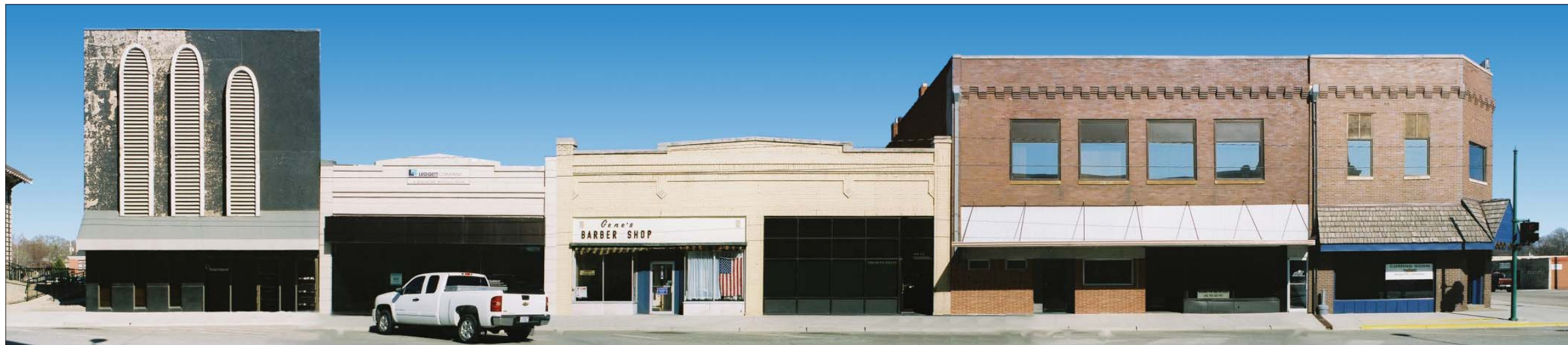
Image 7. Existing Streetscape. The subject building, at left in the photograph, was remodeled some years ago to include reconfiguration of the original second story into a lower-height second story and new third story, with rental housing on both floors. The original tall second story window openings were infilled with masonry, and smaller double hung windows were installed in the reconfigured second and third stories. While the second and third story windows are likely aligned vertically, they may be unevenly spaced (but not too noticeably) in the horizontal dimension on the façade. The remodeling included the addition of an enclosed stairway from the street to the second story on the south side of the building. The false front with three arched, louvered, elements was built full-height across the building's entire front façade, including a wing wall above the enclosed stairway on the south side of the building (see Images 5 and 6).
