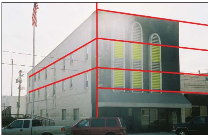
Image 4. Front Façade Window Locations. The locations of the second and third story windows were derived by projecting the lintel lines of the windows on the north wall around the northwest corner of the building and across the front façade. The presumed locations of the windows behind the louvers are marked with yellow shading in the photograph.
