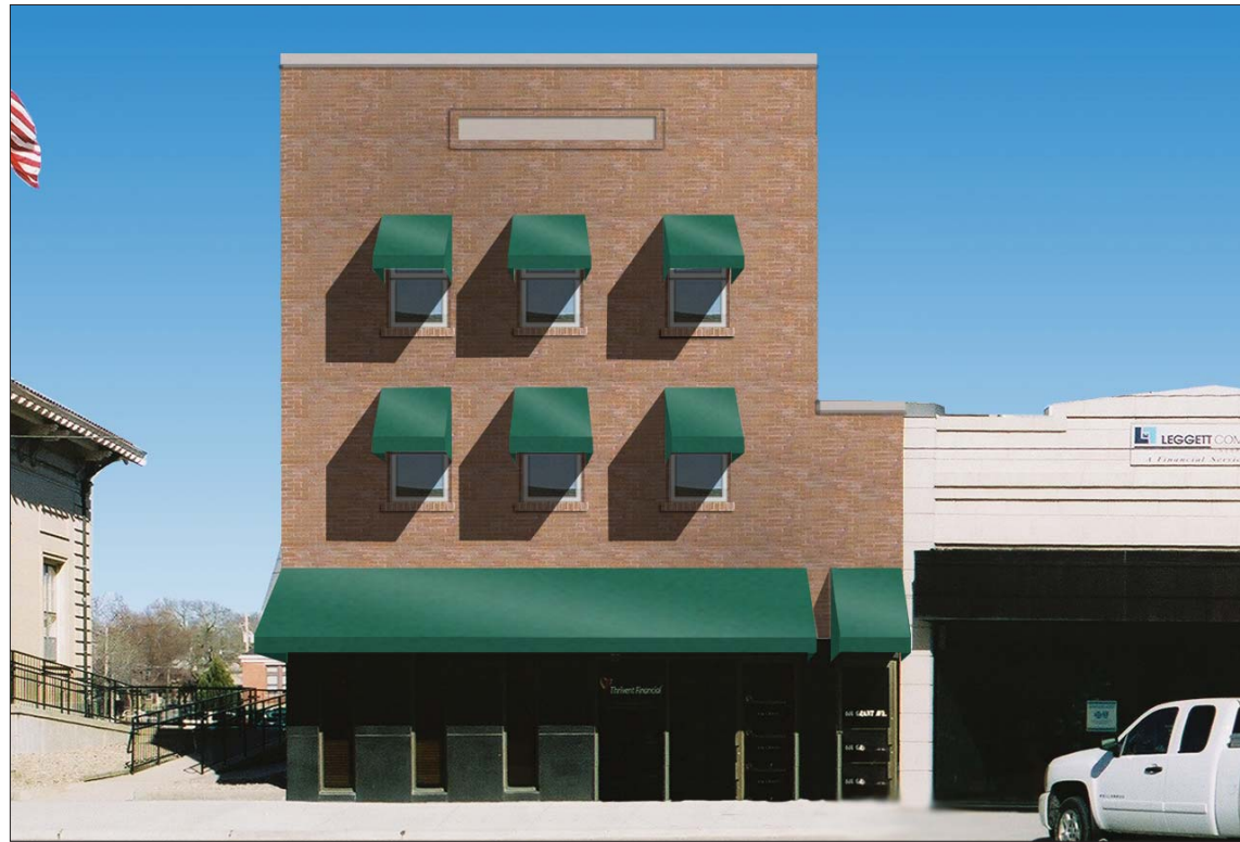
Image 10. Option 1A. The existing false front is replaced with a new facing of thin brick. The wing wall above the enclosed stairway on the south side of the building is removed. A framed building nameplate is integrated with the new brickwork above the third story windows. New double hung windows are installed in existing window openings as necessary. Awnings with Sunbrella's "Erin Green" (#4600) fabric are installed above the second and third story windows, as well as above the storefront on the first floor. A separate awning demarcates the entrance to the enclosed stairway to the upper story housing.
