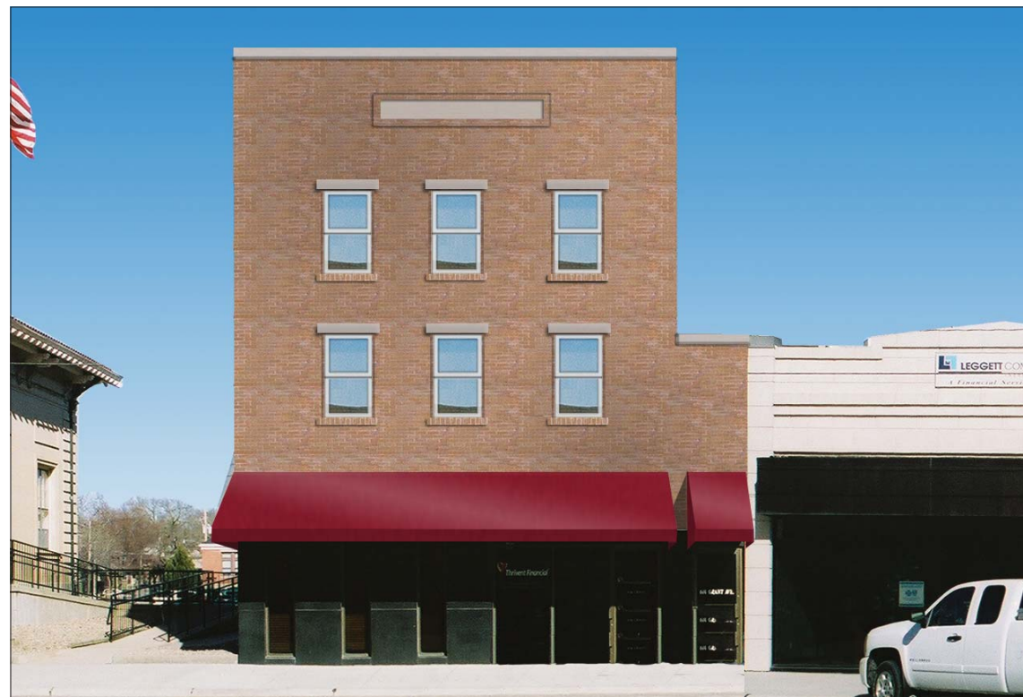
Image 16. Option 1D. Otherwise similar to Option 1C (Image 14), awnings are installed only at the first floor storefront and stairway entrance.
