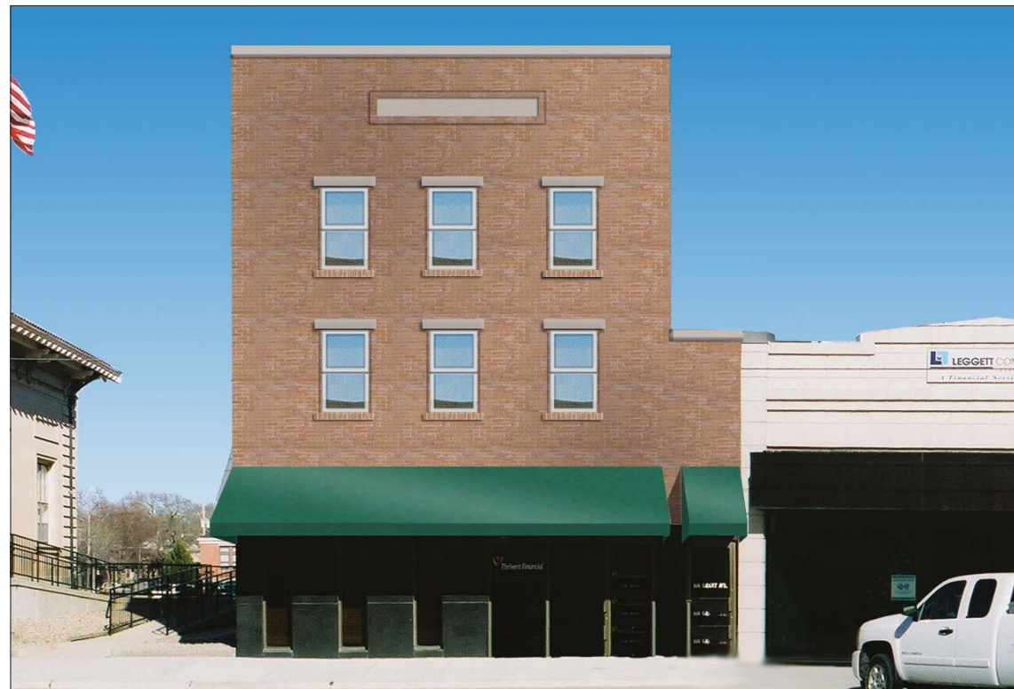
Image 12. Option 1B. Otherwise similar to Option 1A (Image 10), awnings are installed only at the first floor storefront and stairway entrance.
