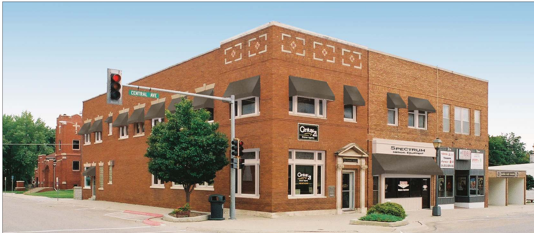
Image 4. Option 1. The corner view shows the effect of new awnings on both the south and west facades.
