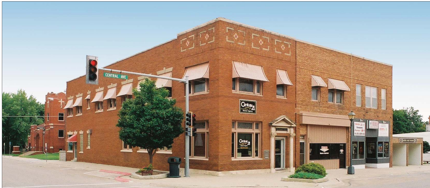
Image 2. Existing Condition. This view from the southwest illustrates how the west and south façades of the corner bank building significantly enhance the streetscapes of Central Avenue and 7th Street. The west façade of the building is punctuated with numerous window openings, especially at the second floor. In contrast to the south window openings, each of the west window openings has a stone lintel with tapered ends and a protruding keystone. All of the second story windows are shaded with metal-slat awnings.
