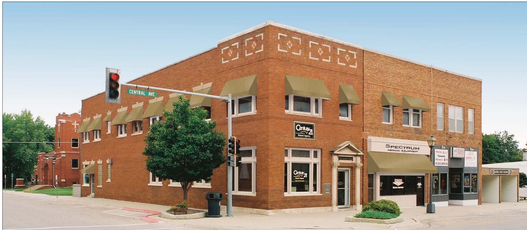
Image 6. Option 2. The corner view shows the effect of new awnings on both the south and west facades.
