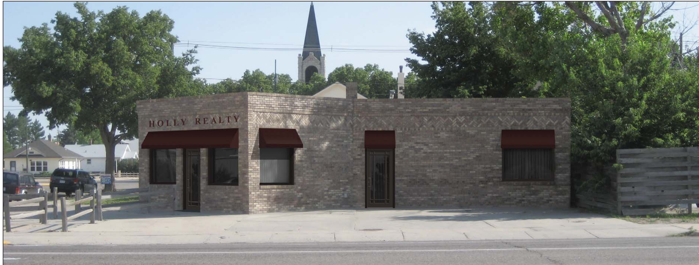
Image 6. Option 2 (North Façade): New bronze architectural detailed commercial storefront doors are installed. Awnings are installed over all windows and doors. The fabric is Sunbrella "True Brown" (#4621). New signage is installed above the main entrance awning. The signage letters are formed plastic, Times New Roman font, with the color to match the awning color.
