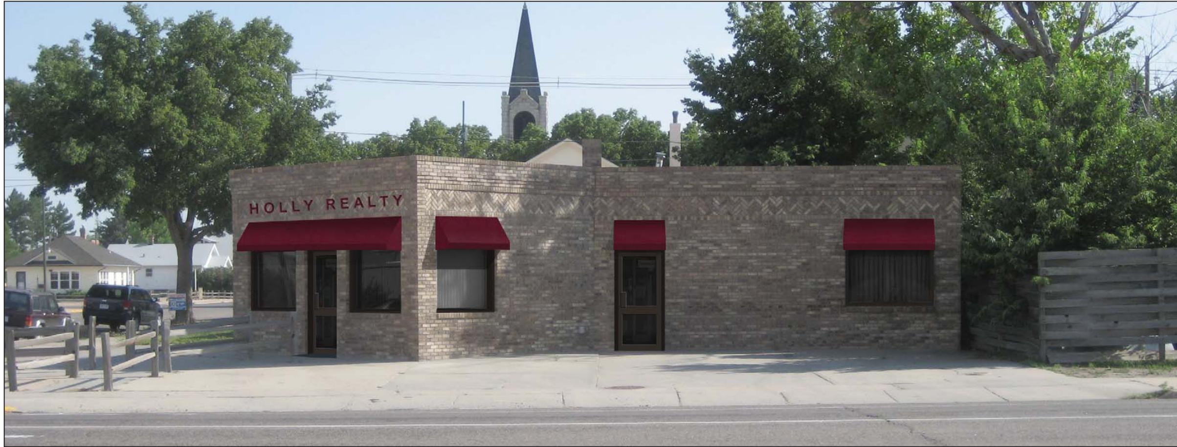
Image 3. Option 1 (North Façade): New bronze standard commercial storefront doors are installed. Awnings are installed over all the windows and doors. The awning fabric is Sunbrella "Burgundy" (#4631). Signage (Arial Bold font) is installed above the main entrance awning.
