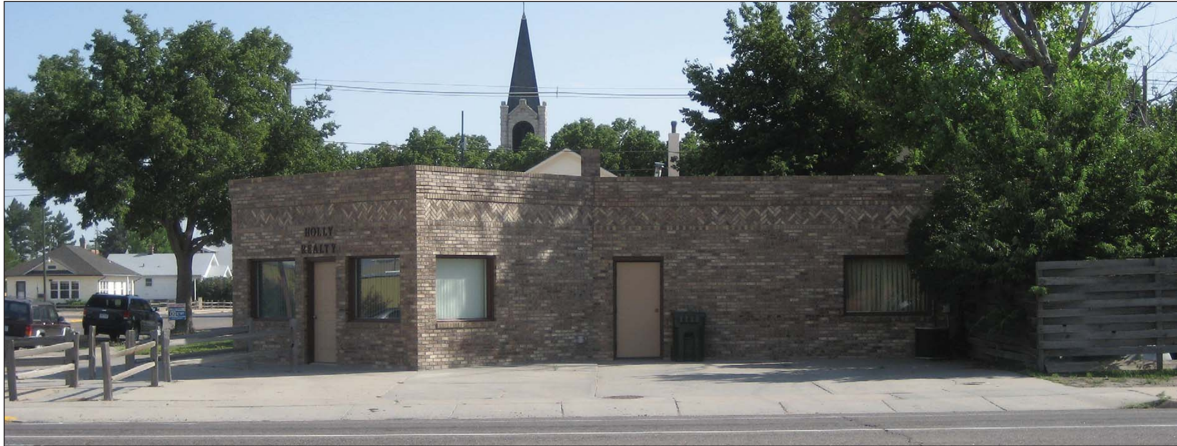
Image 1. Existing Condition (North Façade).
