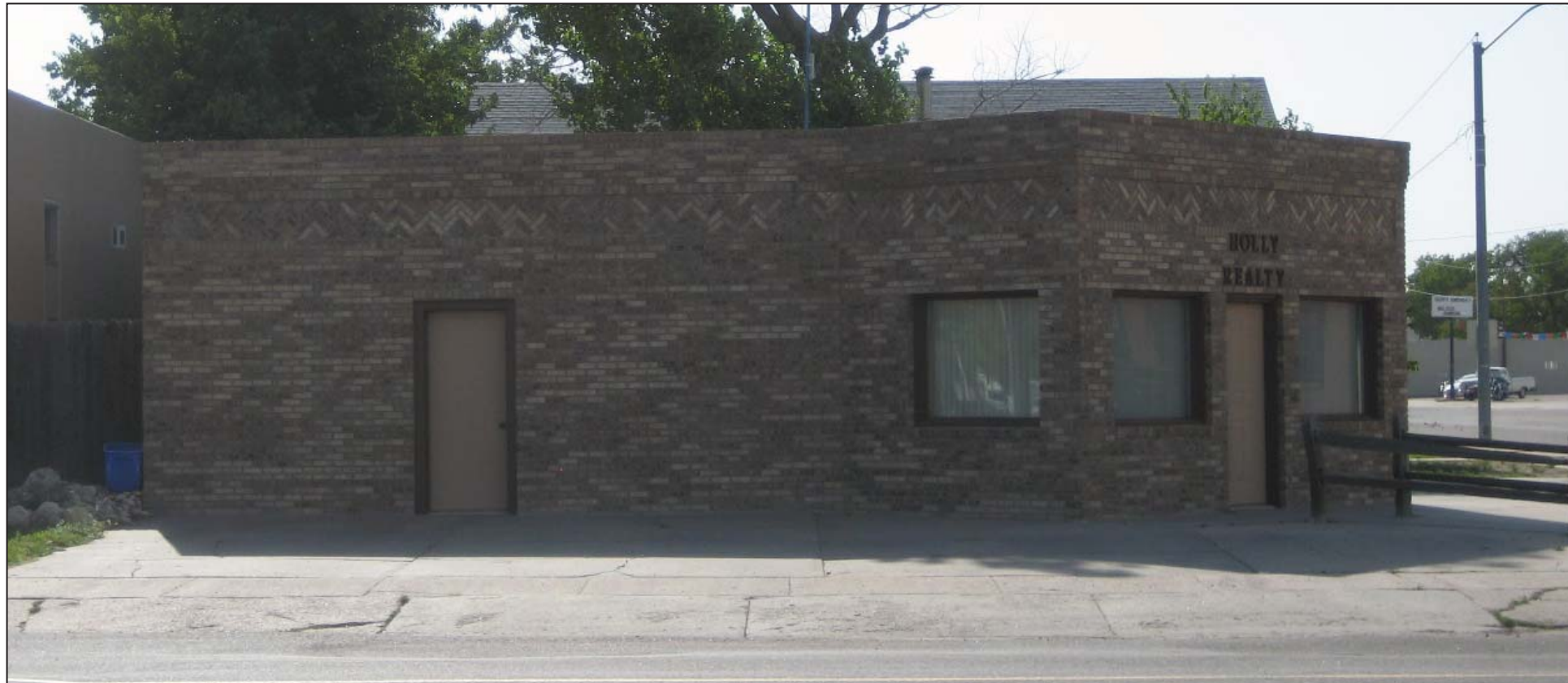
Image 2. Existing Condition (East Façade).
