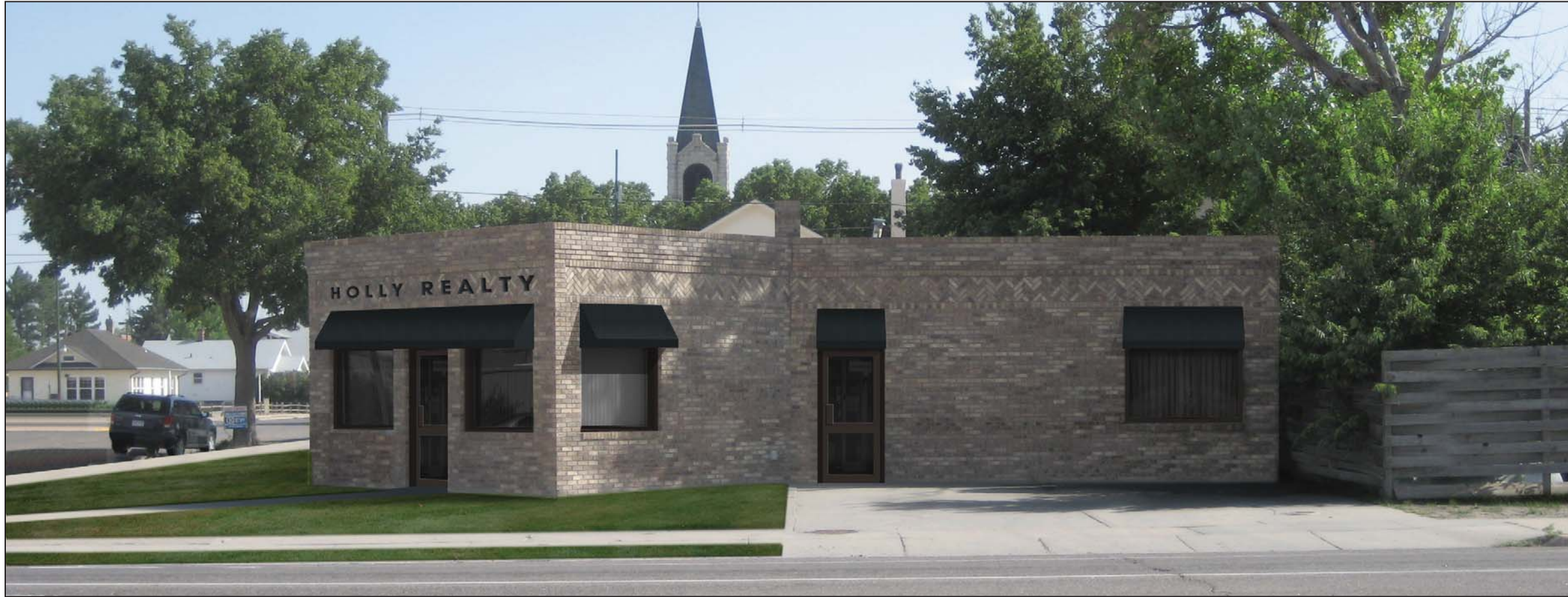
Image 12. Option 4 (North Façade): New bronze commercial storefront doors are installed. Awnings are installed over all windows and doors. The awning fabric is Sunbrella "Alpine" (#4655). The wood fence is removed and replaced with turf to enhance the entry area. Signage (Avant Garde Medium font) is installed above the main entrance awning.
