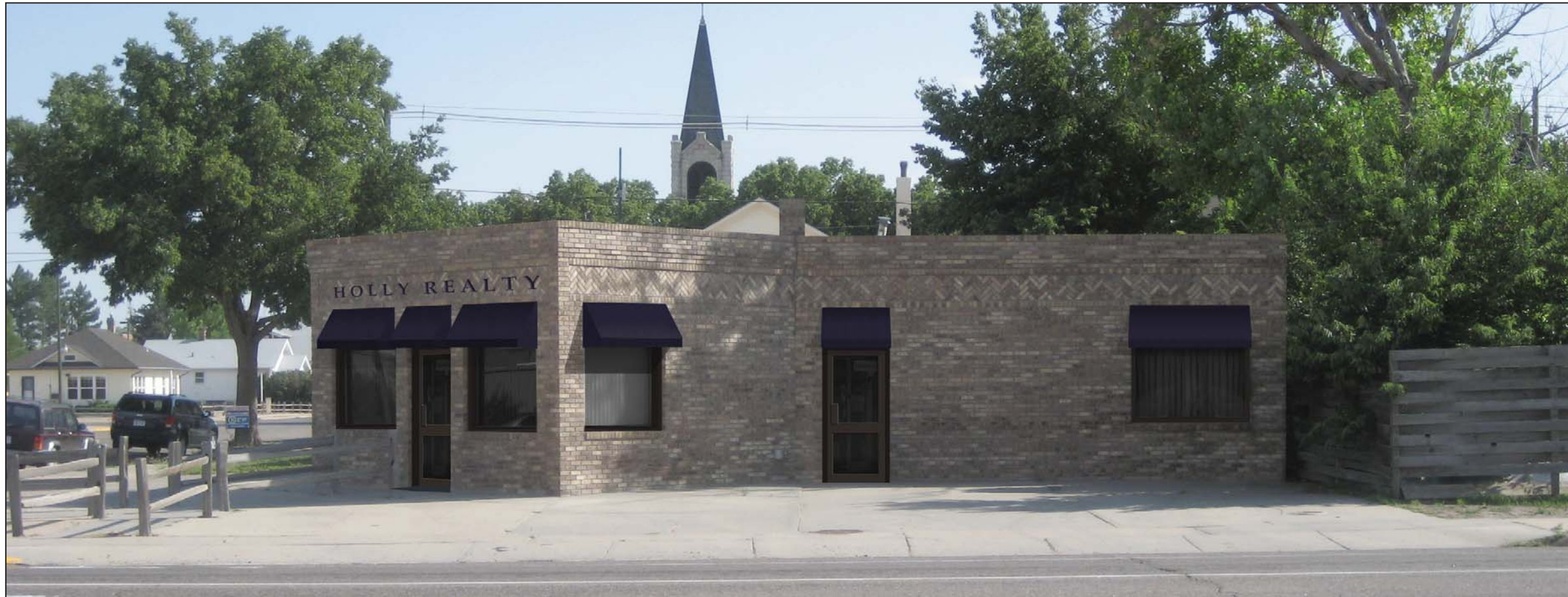
Image 9. Option 3 (North Façade): New bronze commercial storefront doors are installed. Individual awnings are installed over all windows and doors. The awning fabric is Sunbrella "Navy" (#4626). Signage (Palatino font) is installed above the main entrance awnings.
