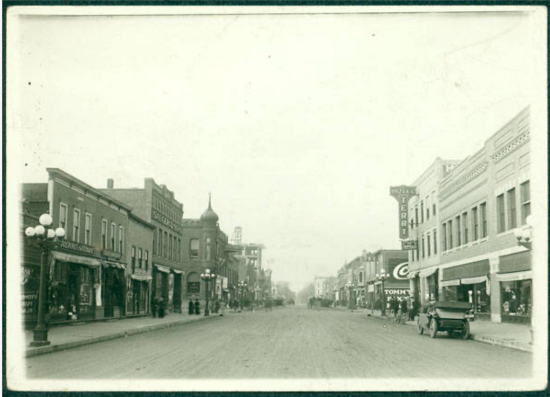
Main Street Photo from about 1913 (Front right shows 338 N Main and part of 330 N Main)
