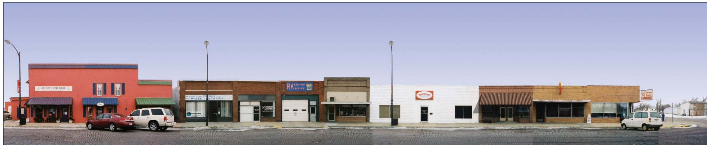
Image 17. Option 5 (Streetscape): This rendering shows Option 5 (Image 15) of the Shear Magic Salon building in the context of the existing block.
