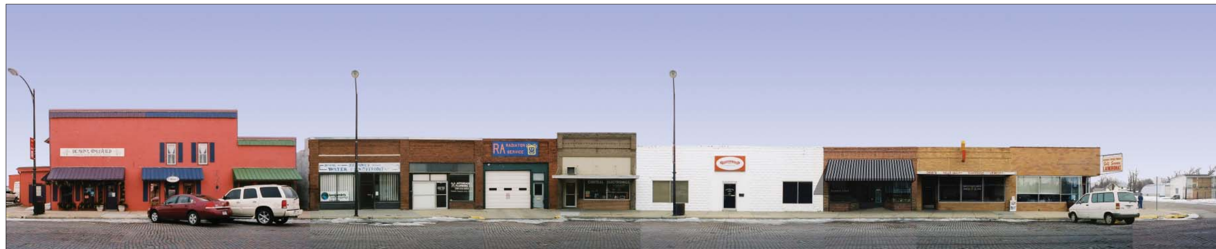
Image 14. Option 4 (Streetscape): This rendering shows Option 4 (Image 12) of the Shear Magic Salon building in the context of the existing block.
