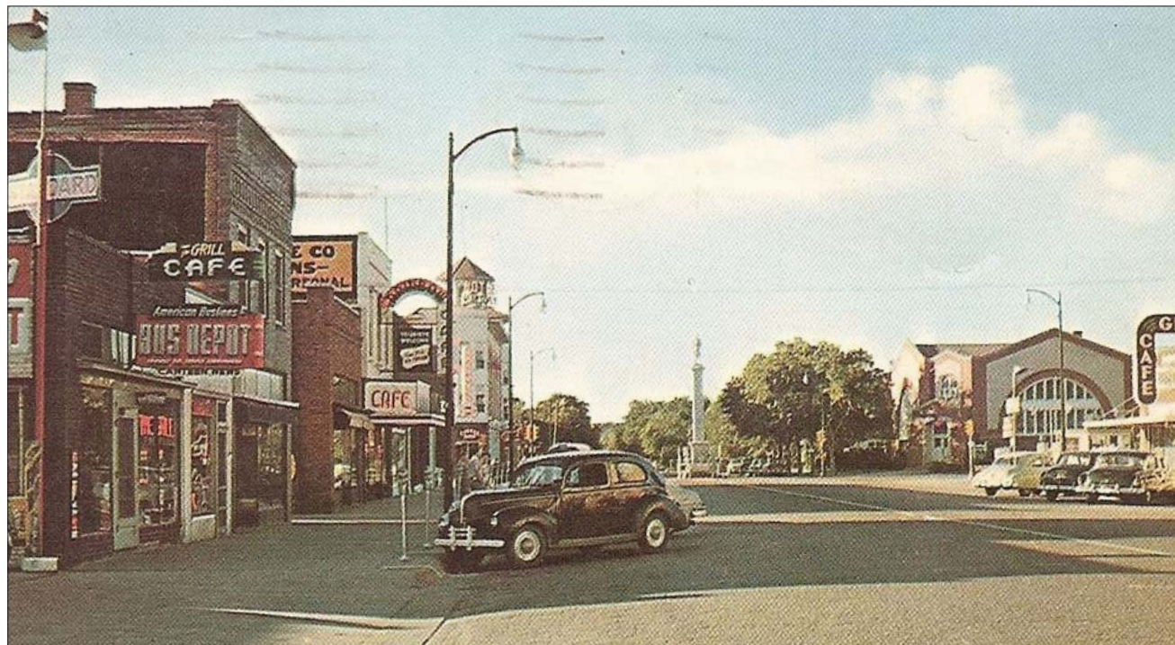
Image 1. Historic Photograph: The facades of the one- and two-story portions of the Helleberg Building are shown at the far left in this historic postcard photograph. A bus depot and a café occupy the one-story portion of the building. Transom windows are evident on both the one-story and two-story portions of the building.
