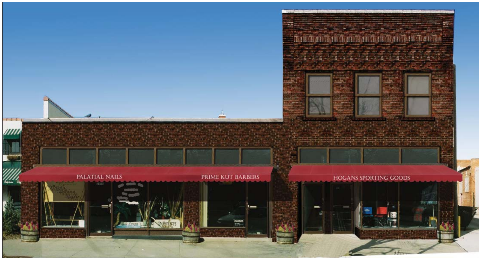
Image 5. Option 1.1: The transom windows on the first floor storefronts are restored, and retractable awnings are installed.
