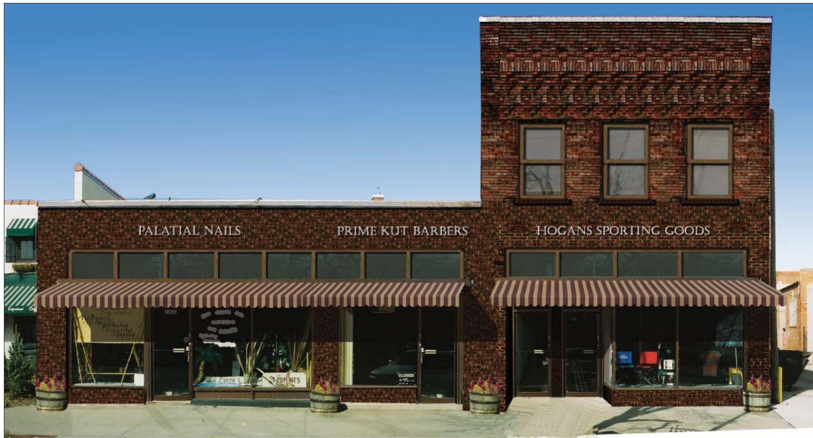
Image 14. Option 4.1: The transom windows on the first floor storefronts are restored, and retractable awnings are installed.
