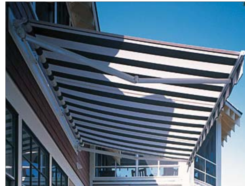
Image 3. Retractable Awning: This example installation of a retractable awning—proposed in the design options presented on the following sheets—illustrates its extended position, as well as its typical mounting condition on the building façade (source: www.sunbrella.com).
