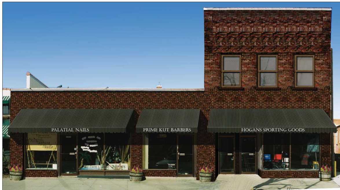
Image 12. Option 3.2: Three conventional fixed awnings are installed on the storefronts to demarcate the three stores in the building.
