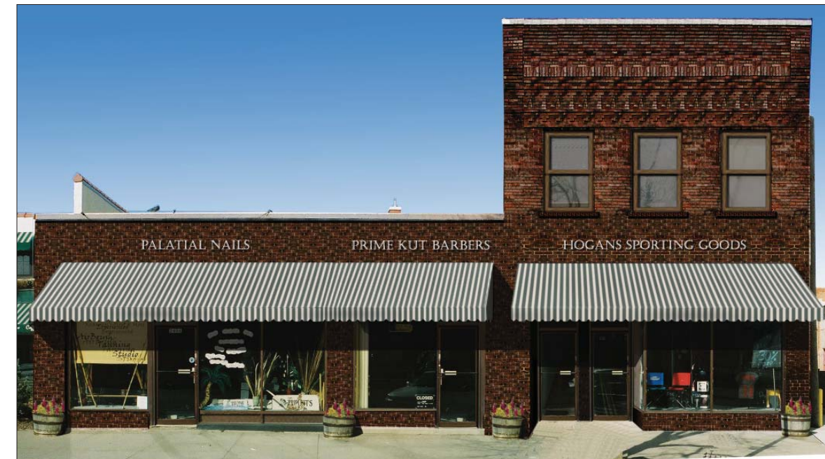
Image 19. Option 5.3: Two conventional fixed awnings are installed on the storefronts, one on the one-story portion of the building, and one on the two-story portion of the building.
