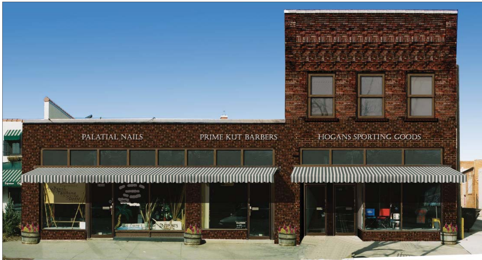
Image 17. Option 5.1: The transom windows on the first floor storefronts are restored, and retractable awnings are installed.
