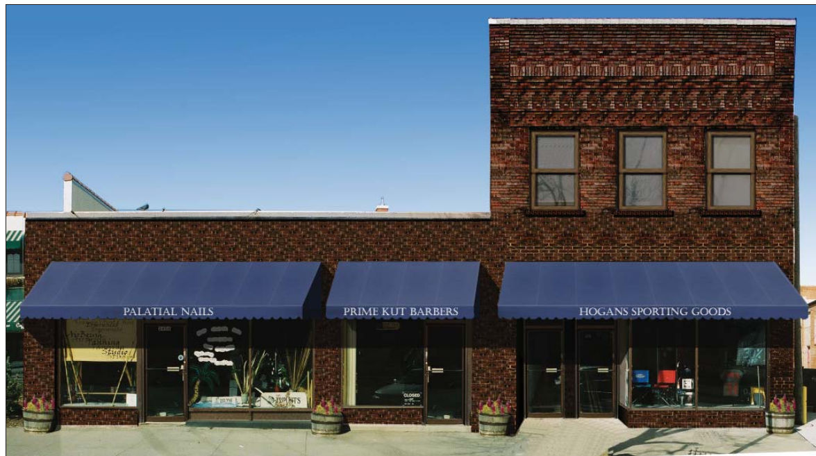
Image 9. Option 2.2: Three conventional fixed awnings are installed on the storefronts to demarcate the three stores in the building.
