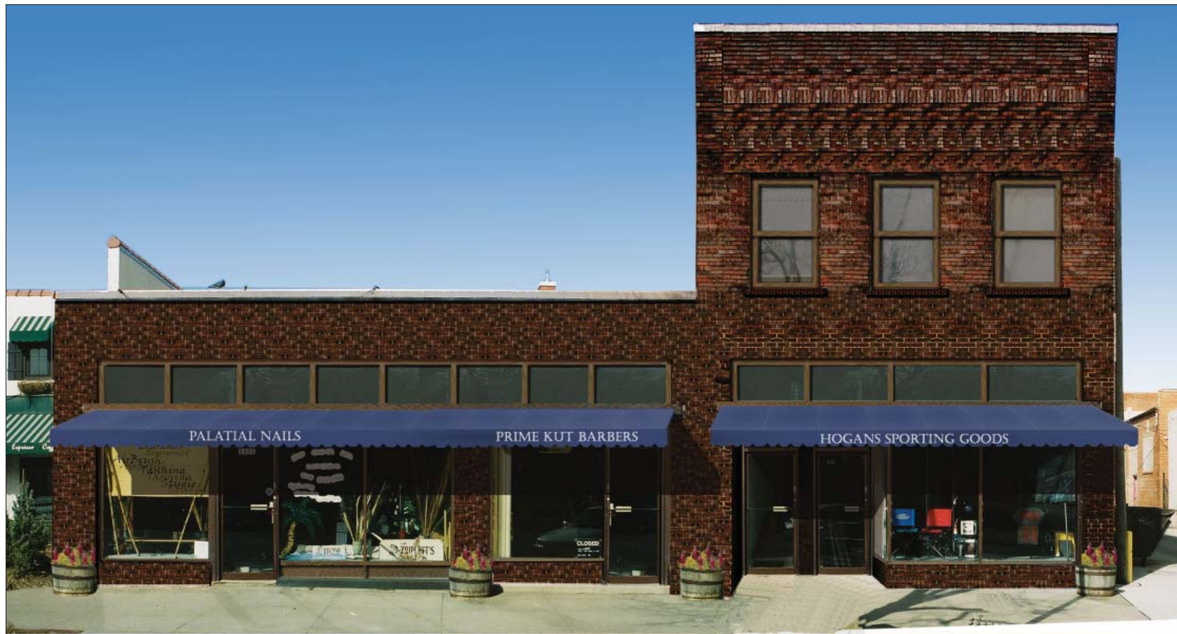
Image 8. Option 2.1: The transom windows on the first floor storefronts are restored, and retractable awnings are installed.
