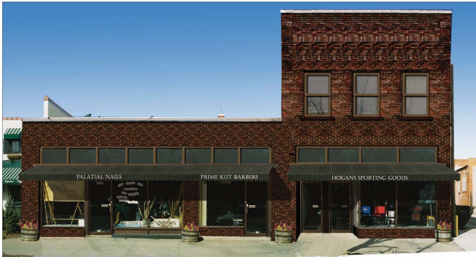
Image 11. Option 3.1: The transom windows on the first floor storefronts are restored, and retractable awnings are installed.
