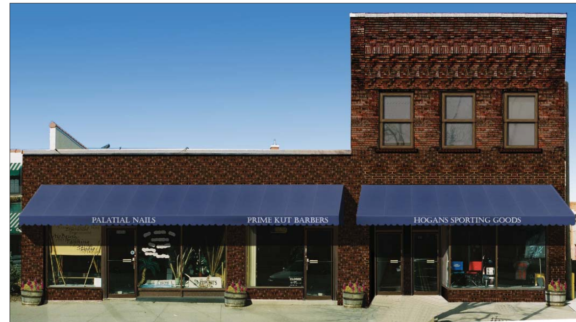
Image 10. Option 2.3: Two conventional fixed awnings are installed on the storefronts, one on the one-story portion of the building, and one on the two-story portion of the building.
