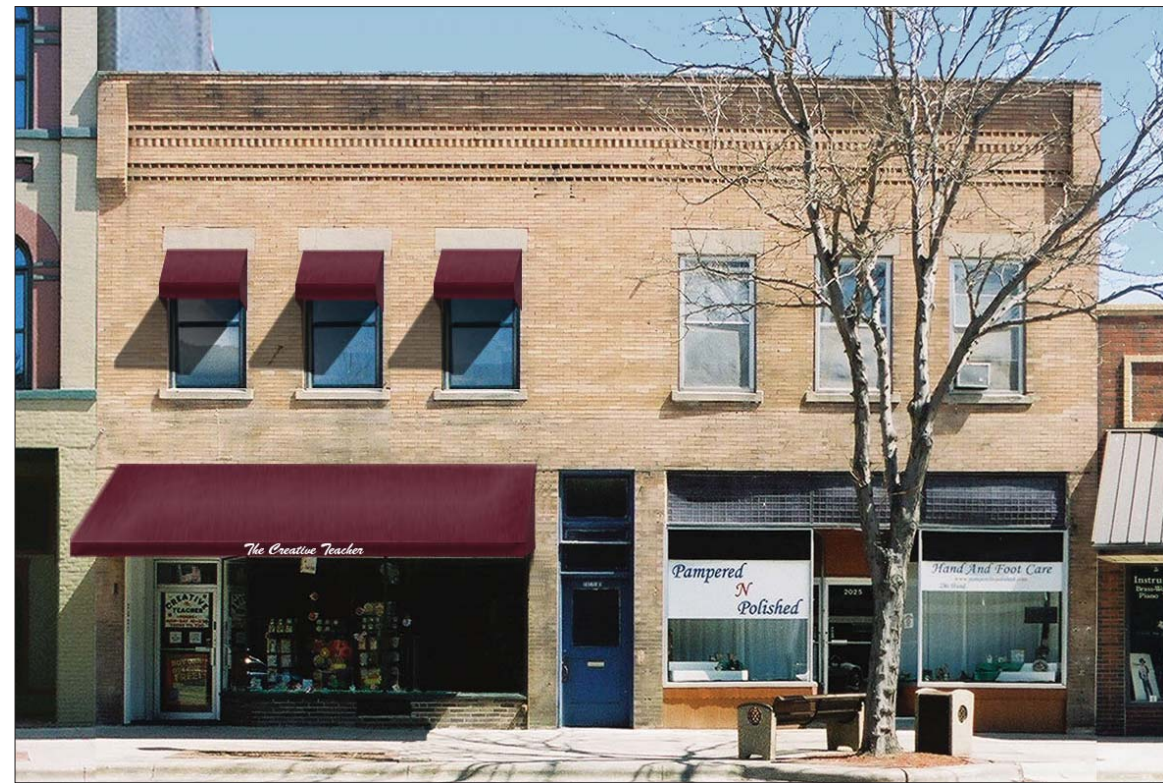
Image 16. Option 3.1: A full-width fixed awning is installed above the storefront door and display window, shielding the transom windows. Signage is appliquéd to the awning valance. Three fixed awnings are installed on the new bronze-colored metal double hung windows on the second story.
