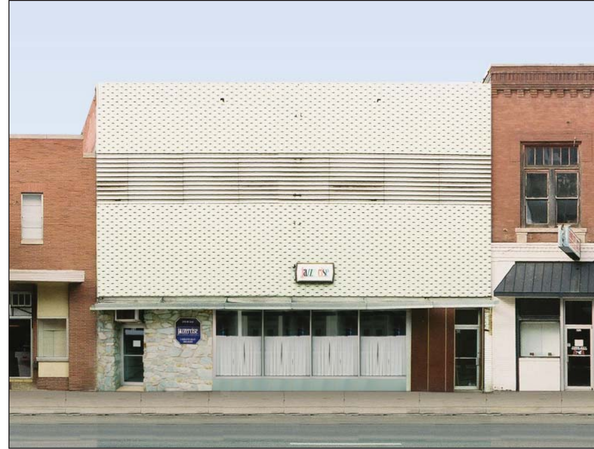
Image 2. Existing Condition. In recent years a metal false front was installed over the upper portion of the Majestic Theatre building façade. The lower façade was reconfigured to address recent building needs. Because the false front remains intact, the condition of the original façade is unknown, although it appears that the decorative vertical extensions of the parapet wall have been removed.
