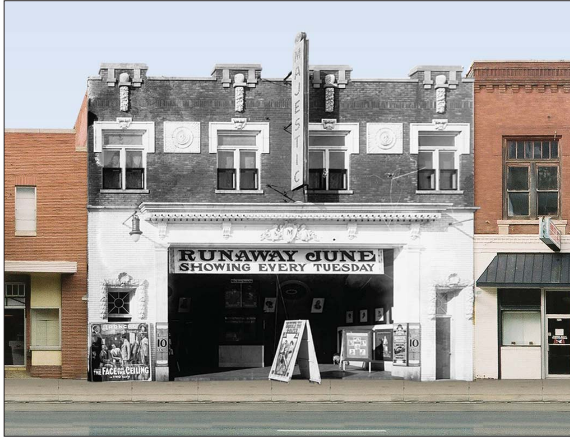
Image 1. Historic/ Present Day Photomontage. A historic 1915 photo of the old Majestic Theatre is superimposed on a photograph of the current block façade. The early photograph of the Majestic Theatre building, including second story window hoods, coping, cornice, medallions, etc., shows extensive terra-cotta ornamentation.
