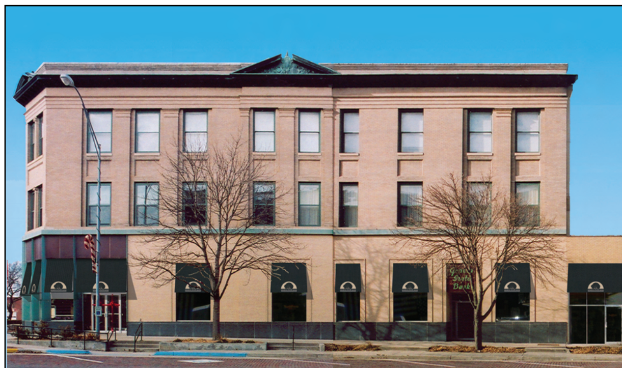
Image 9. Option 2 (East Facade): The Geneva State Bank logo is applied to each awning. Awnings with Sunbrella "Alpine" (style #4655) fabric are installed on the first floor windows of the existing bank facade.
