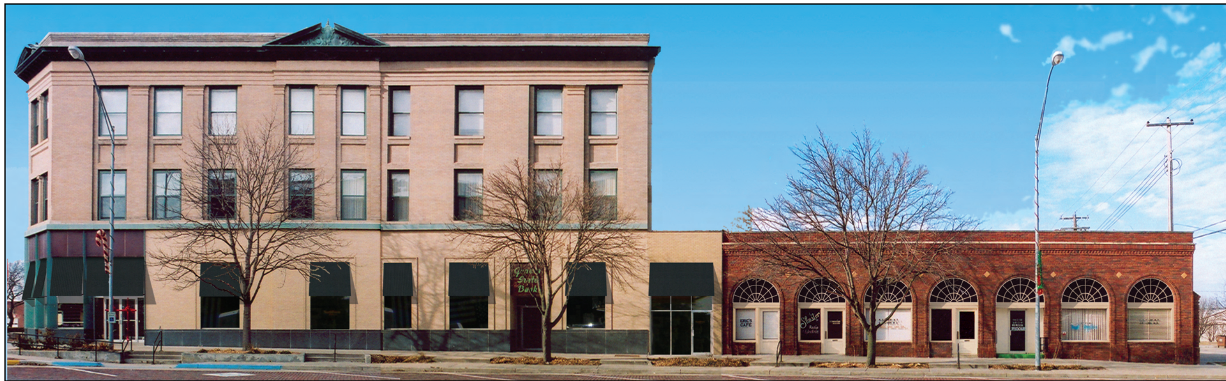
Image 7. Option 1 (East Facade): Awnings with Sunbrella "Alpine" (style #4655) fabric are added to the first floor windows on the existing bank facade. This option includes opening the fanlights in the Ashby Building and painting all doors, window and door frames, and muntins to match the stone veneer on the main bank building.
