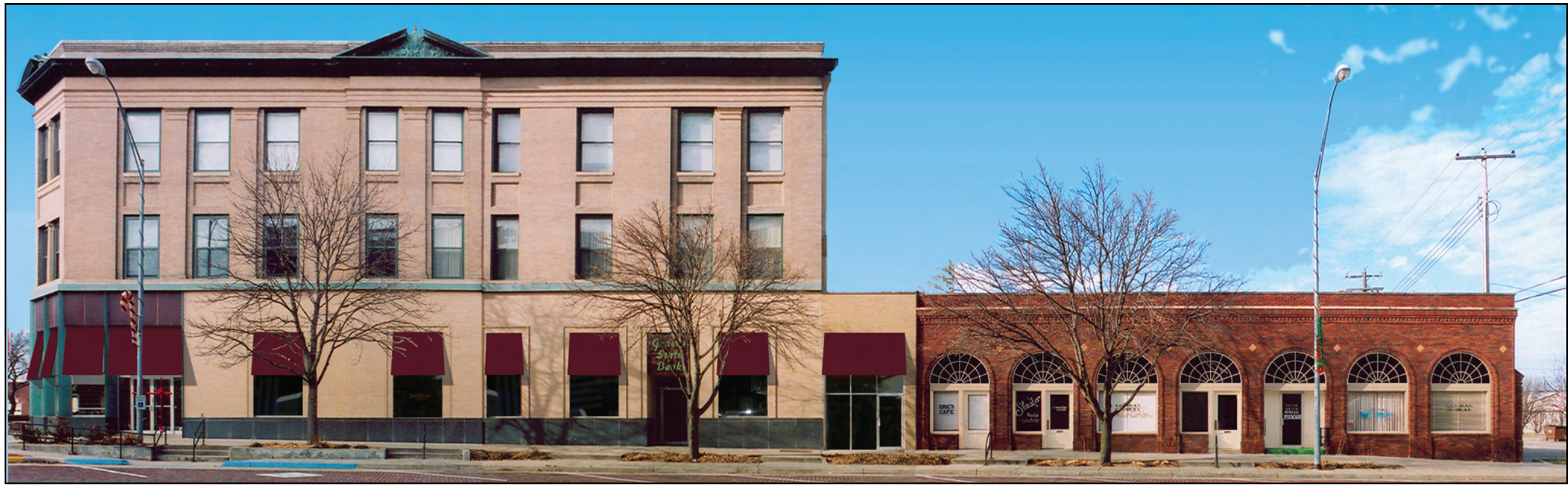
Image 15. Option 5 (East Facade): Awnings with Sunbrella "Burgundy" (style #4631) fabric are added to the first floor windows on the existing North 9th Street and G Street bank facades. This option includes opening the fanlights in the Ashby Building (right). Also, the doors, window and door frames, and window muntins on the Ashby Building are painted to match the stone veneer on the main bank building.
