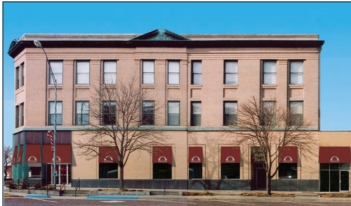
Image 13. Option 4 (East Facade): This image shows the Geneva State Bank logo on each awning. Awnings with Sunbrella "Terra Cotta" (style #4622) fabric have been added to the windows on the existing bank facade.
