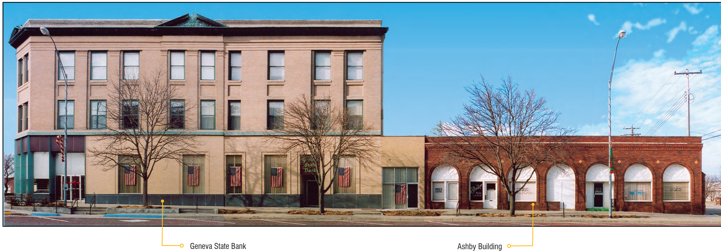
Image 4. The existing condition of the east facade of the three-story Geneva State Bank (left) and the adjoining one-story red brick Ashby Building to the north (right) is shown in this photograph. The first floor of the 1906 bank building was extensively remodeled on the interior and exterior in 1961 (compare with Images 1 and 2). The intricate detailing of the fanlights in the Ashby Building has been obliterated by white paint which covers the glass and muntins.
