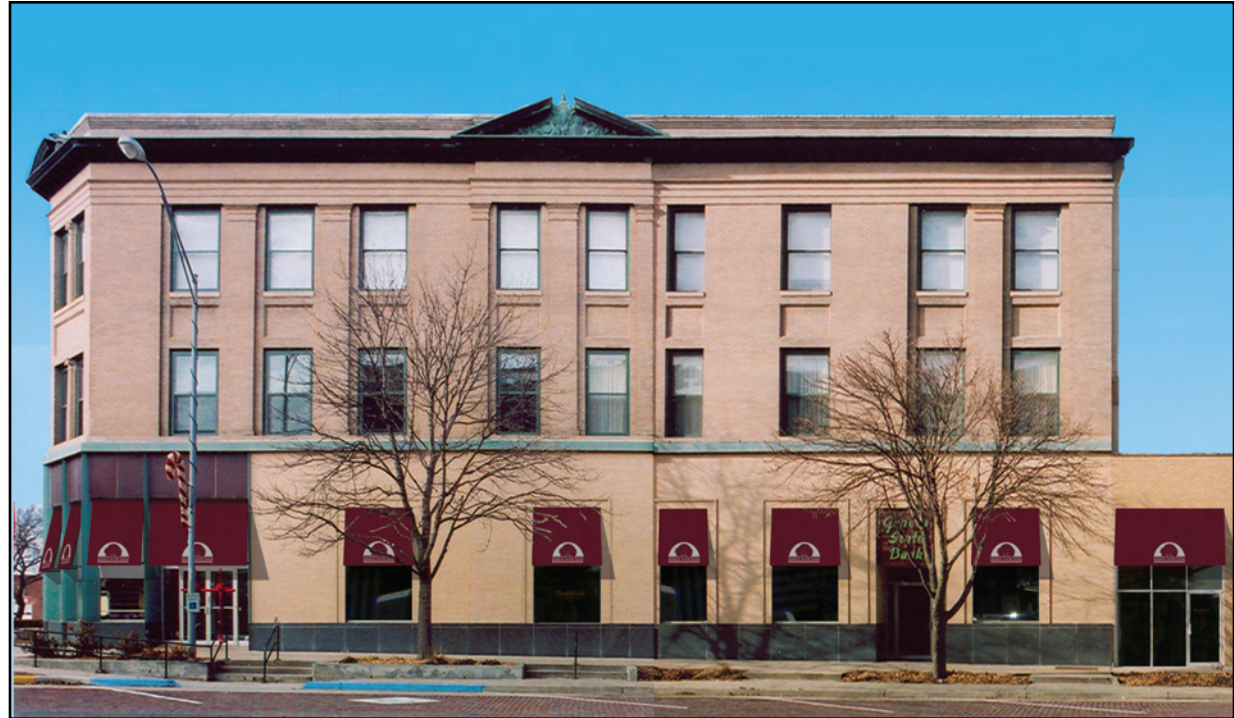
Image 17. Option 6 (East Facade): The Geneva State Bank logo is applied to each awning. Awnings with Sunbrella "Burgundy" (style #4631) fabric are installed on the first floor windows of the existing bank facade.
