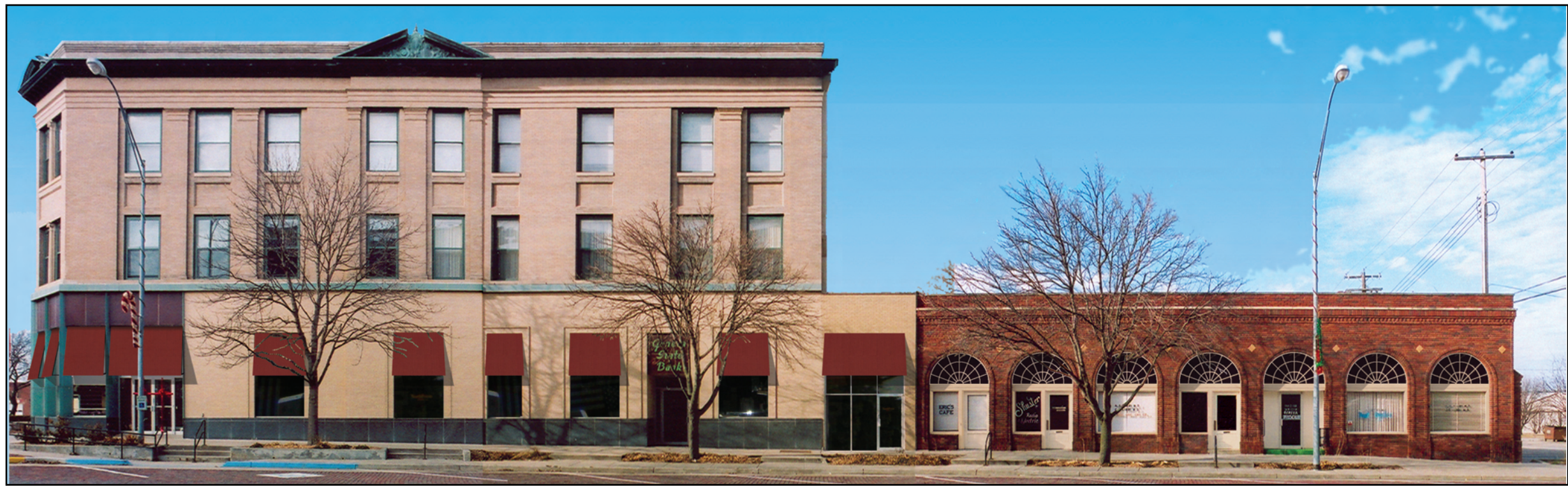
Image 11. Option 3 (East Facade): Awnings with Sunbrella "Terra Cotta" (style #4622) fabric are added to the windows on the existing bank facade. This option includes opening the fanlights in the Ashby Building and painting all doors, window and door frames, and window muntins to match the stone veneer on the main bank building.
