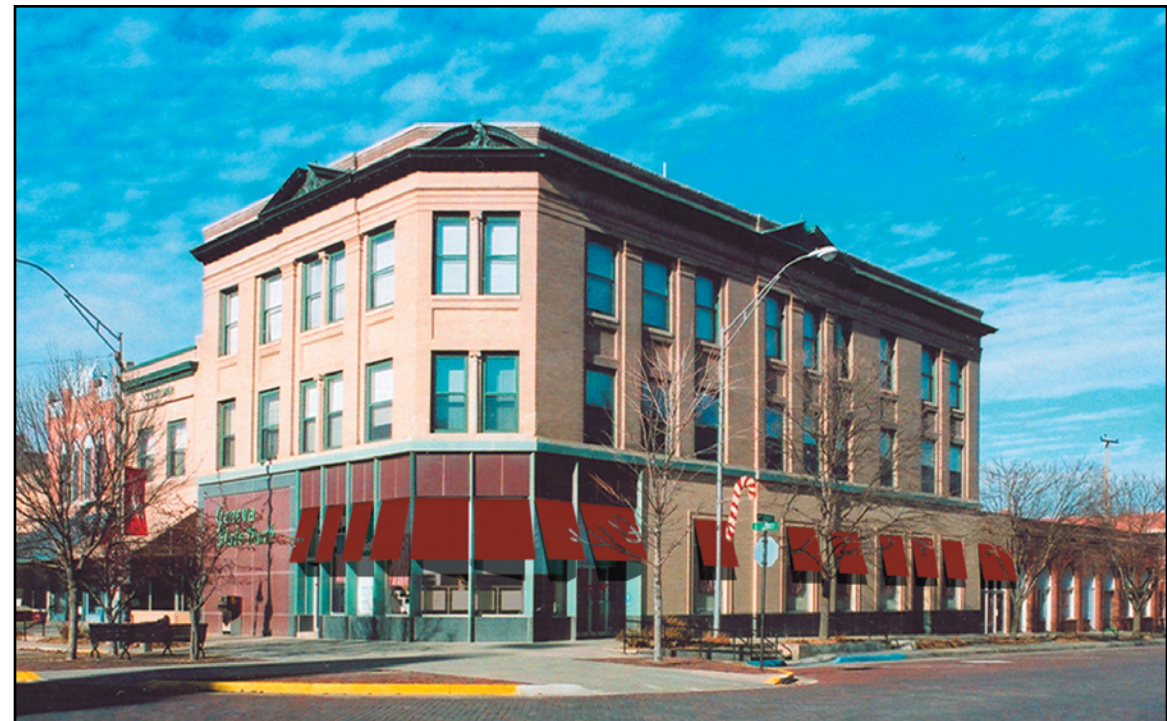
Image 14. Option 3 (G and North 9th): Awnings with Sunbrella "Terra Cotta" (style #4622) fabric are installed on the first floor windows of the 1961 facade of the bank.
