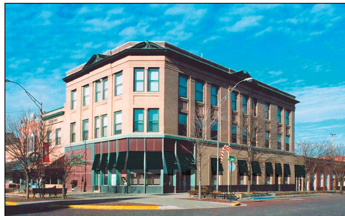
Image 10. Option 1 (G and North 9th): Awnings with Sunbrella "Alpine" (style #4655) fabric are installed on the first floor windows of the 1961 remodeled facade of the bank.
