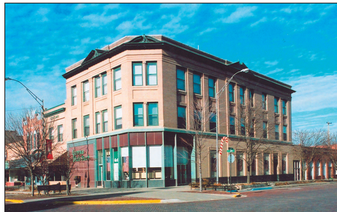
Image 6. The existing condition of the Geneva State Bank is shown in this corner view, looking northwest at the intersection of G and North 9th Streets. The effect of the 1961 first floor remodeling of the 1906 building is illustrated (compare with Image 1).
