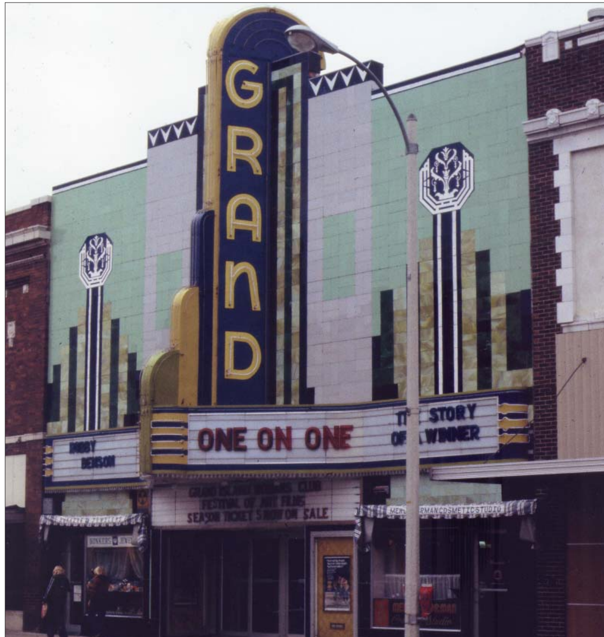
Image 3. Historic Photograph, 1977: Signage and marquee alterations can again be observed when compared to Image 2, as well as changes to the lower-facade.
