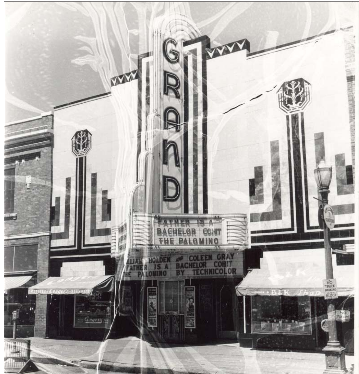
Image 2. Historic Photograph, c. 1940: The Grand Theatre was subjected to modification just a few years after its opening.
