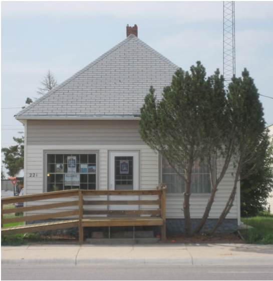
existing condition with tree
