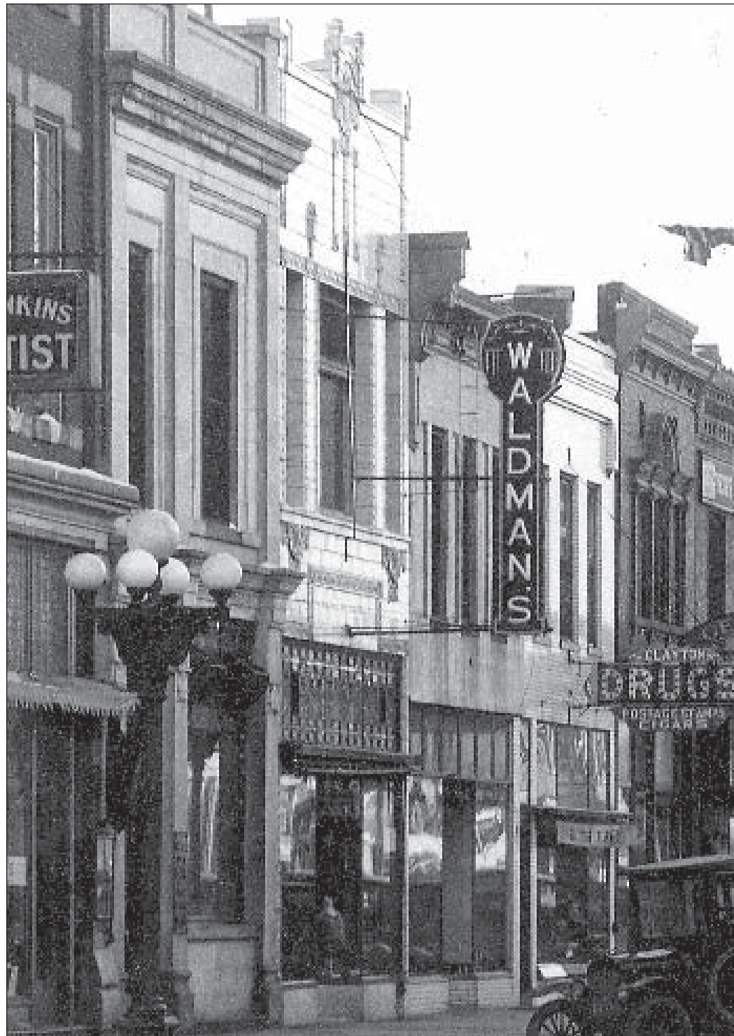
Image 1: Historical Photograph. In this early photograph of the present Connie Swanson Photography building, all parts of the original façade—including second story windows; terra-cotta coping, cornice, sills, and accent pieces; full-width transom window; and storefront windows—are intact. The building is shown to have been a Waldman's store.
