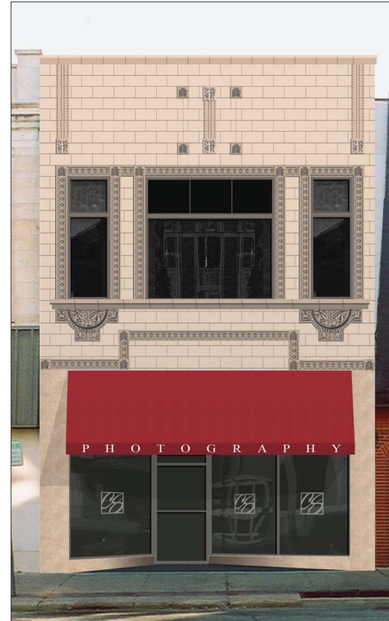
Image 27: Option 4. Otherwise similar to Image 26, this proposal replaces damaged or lost terra-cotta units on the lower portion of the building with porcelain tile, a sample of which is depicted in Image 17.
