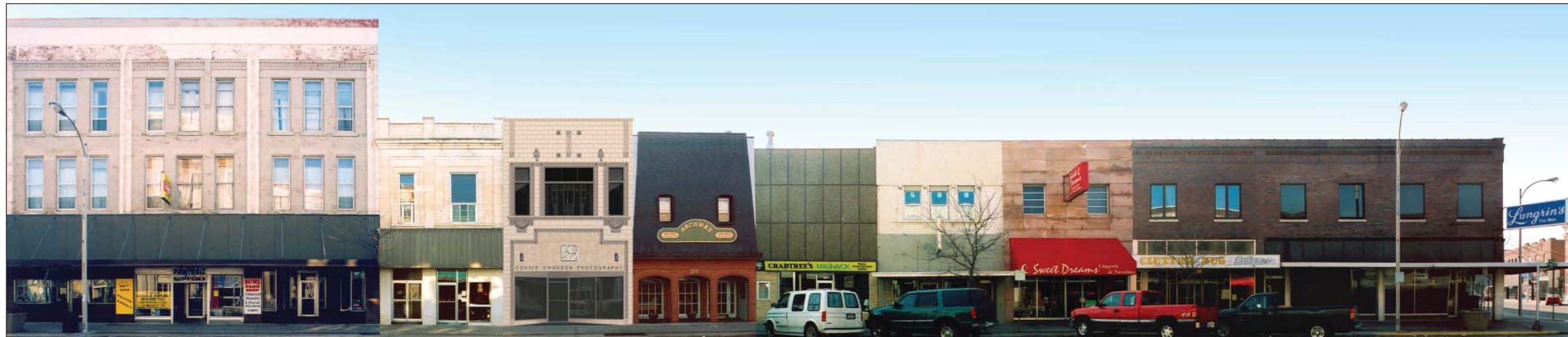
Image 8: Option 2. This view shows the north-facing building frontage of the 200 block of West 3rd Street if Option 2 (Images 18-20) is utilized for the Connie Swanson Photography building.
