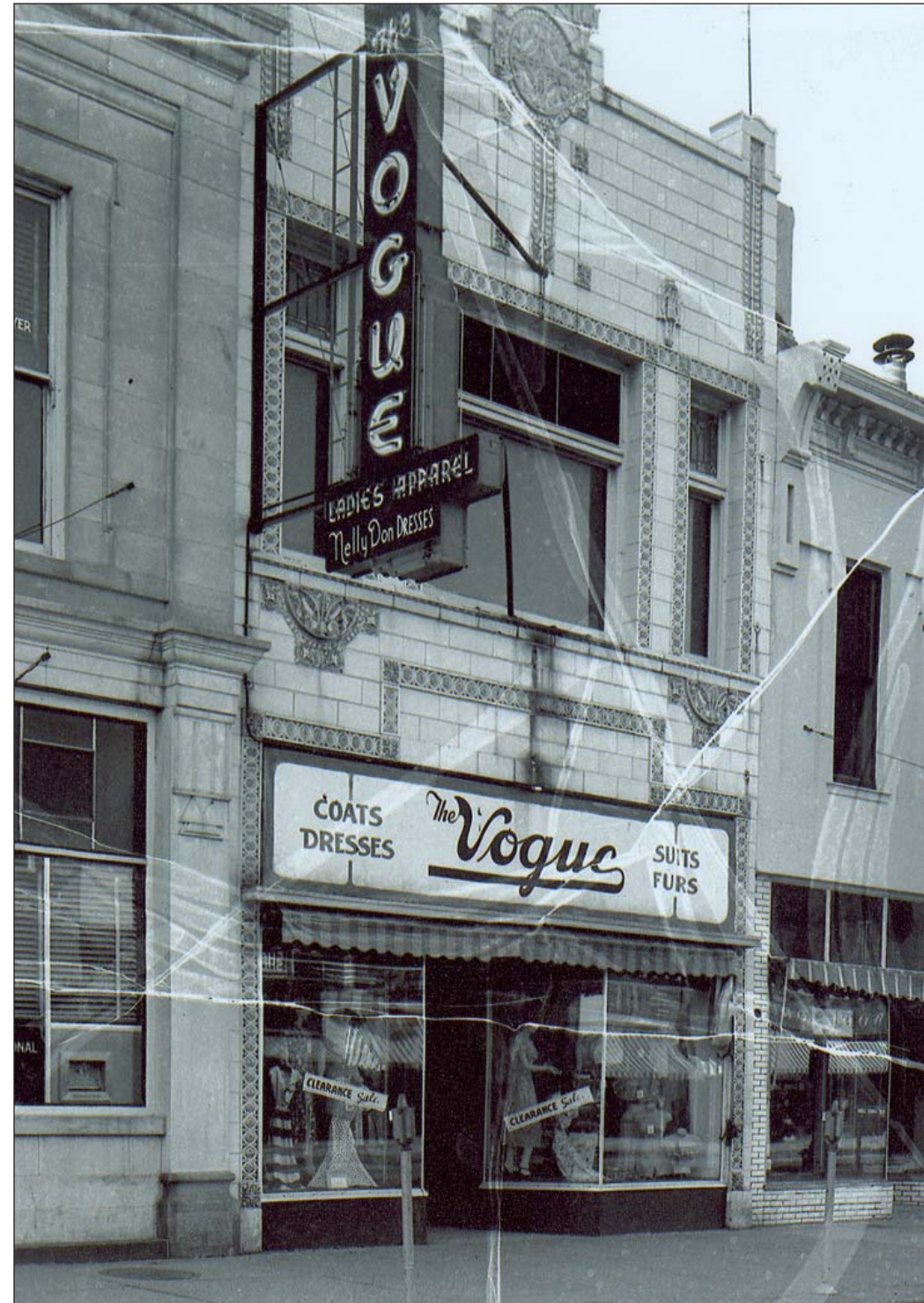
Image 2: Historical Photograph. In this photograph, the Connie Swanson Photography building is shown to have been the Vogue Ladies Apparel Store. The transom window has been covered with a "Vogue" signboard. Previous signage has been removed and some damage to the terra-cotta is evident. The storefront has also been modified.
