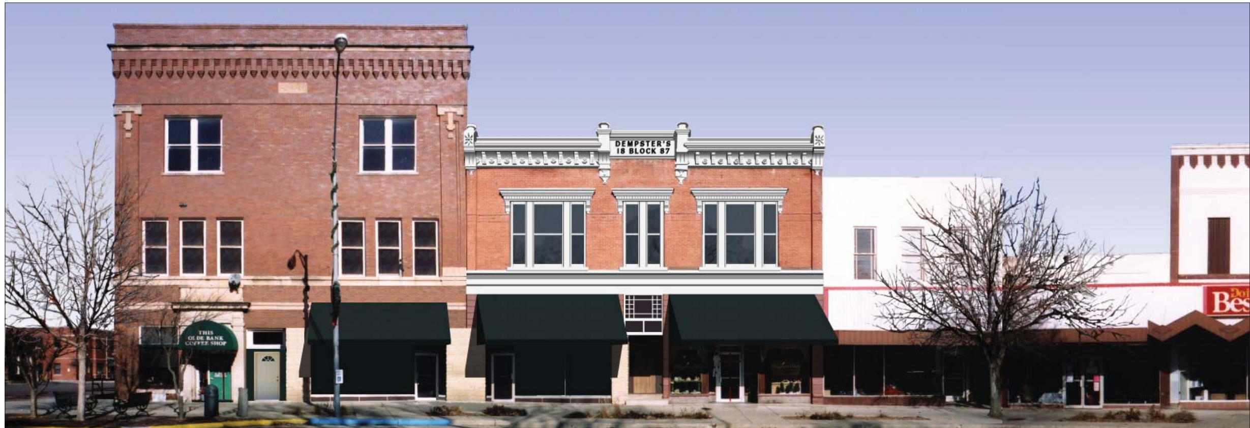
Image 7. Option 3 (South Facade): The existing awning/canopy is removed from both the F&M Building and Dempster's Block and is replaced with three awnings (fabric is Sunbrella's "Alpine" #4655). The removal of the awning/canopy will presumably reveal transom windows on both buildings, as well as cast iron piers on the Dempster's Block, extending to the second floor level. New second floor windows on the Dempster's Block are installed, and the architectural features including the window frames, hoods and cornice are painted white. All of the existing signage at the second floor level is removed.
