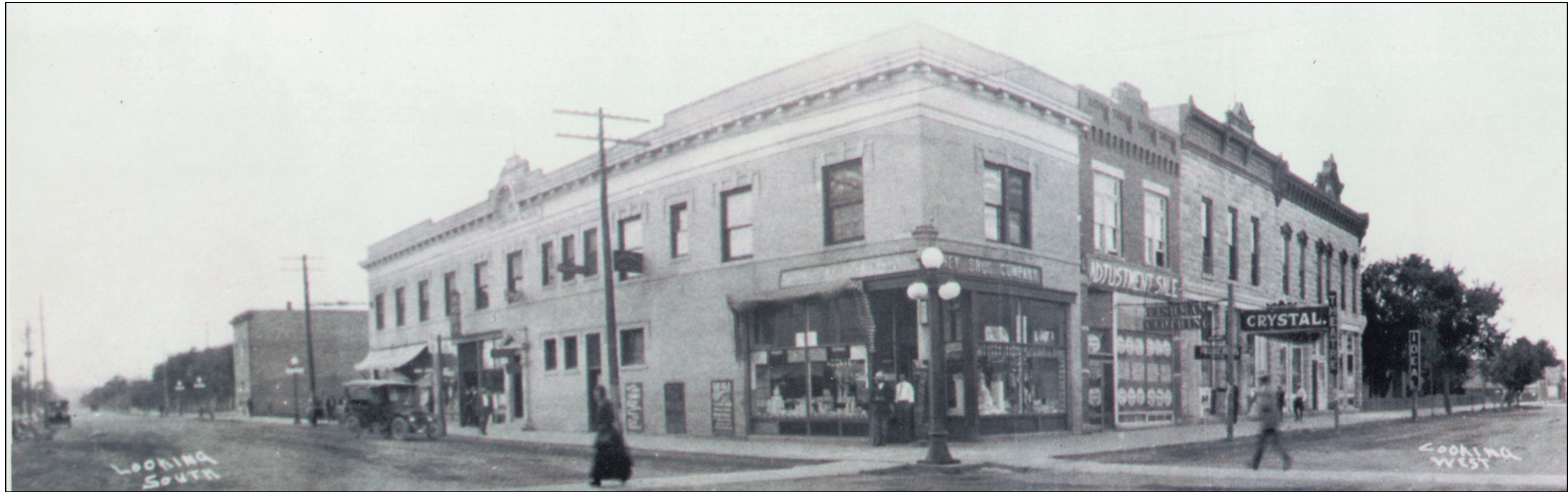
Image 1. This historical photograph shows the Cleburne-McIntosh Block, on the southwest corner of 10th Avenue and Illinois Street, not long after it was constructed in 1908. The north and east facades are finished with pressed-face brick and Bedford limestone. The first floor was originally divided into three retail spaces: (1) Sidney Drug Company in the north portion, (2) a stationery store; and (3) a dry
