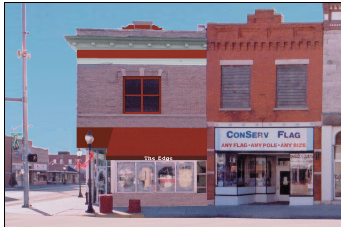
Image 9. Option 2: This image depicts changes similar to those proposed for the east block face, such as awnings, cornice and accent paint, and removal of the corner sign (see image 4).
