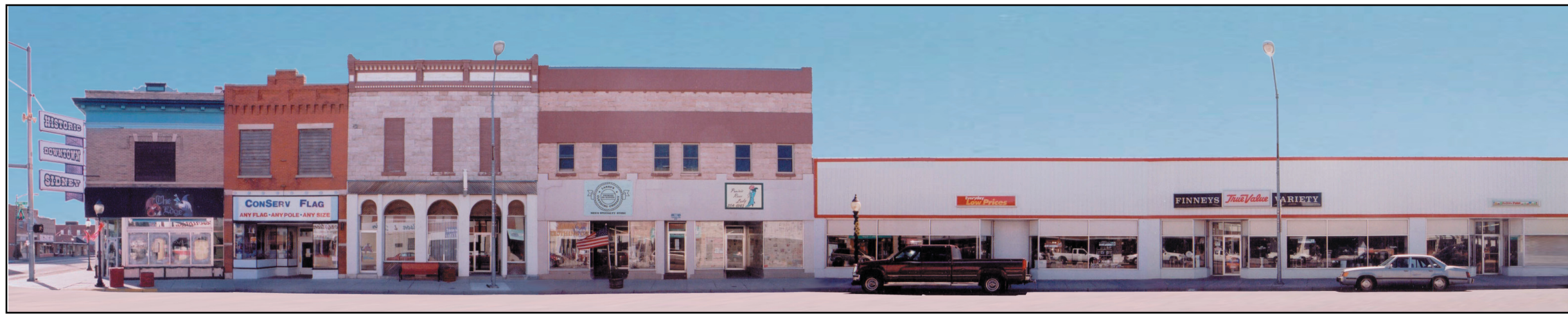
Image 7. The existing condition of the north Illinois Street elevation of the Cleburne-Gaston Building (far left) shows that the original facade has been severely compromised by alterations, including the application of corrugated and textured panels to a large part of the facade.
