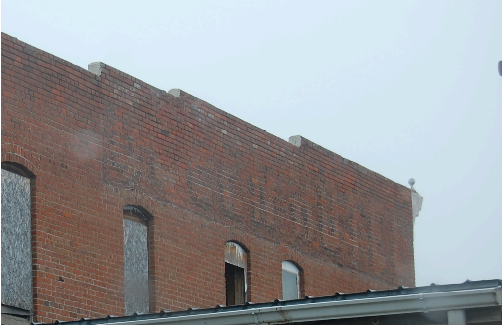
"Queen Hotel" is written on the old mural on the south side of the building.
