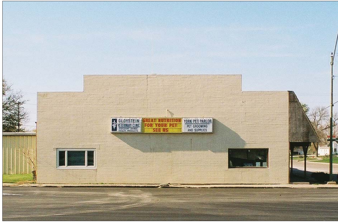
Image 1. Existing Condition. The east façade of the building, facing Lincoln Avenue, is the original brick-faced front of the building. In 1986 the building was remodeled. The east entrance was removed and infilled with masonry. The east brick wall is now painted. An illuminated box sign is mounted on the exterior wall.
