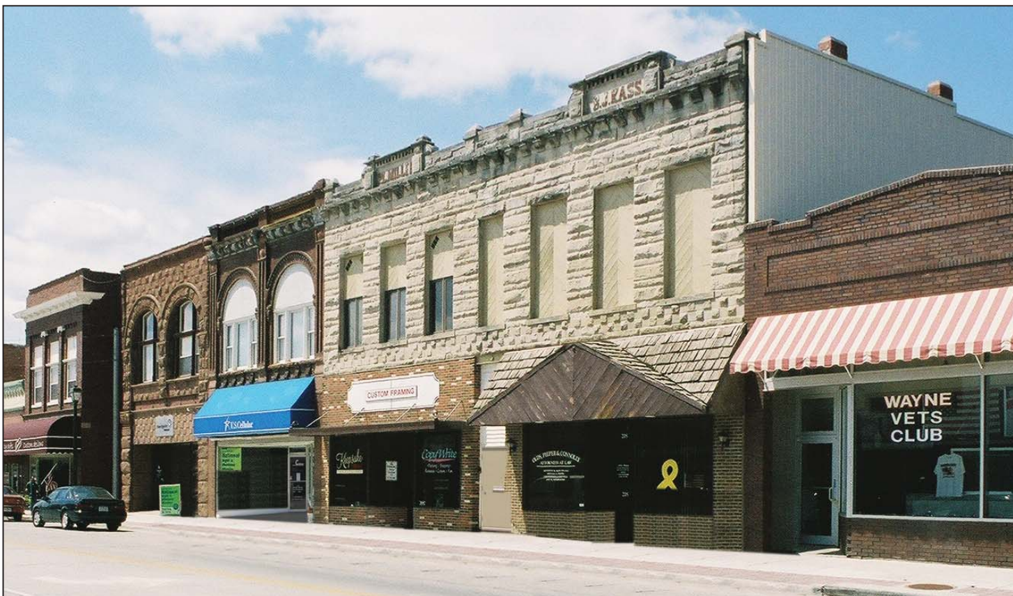
Image 2. Existing Condition. The thin brick and wood gabled awning will be removed. The thin brick is to be replaced with a combination of stucco and porcelain tile. The wood gabled awning is to be replaced with a fabric awning.
