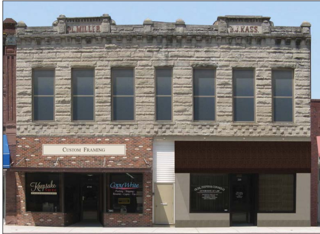
Image 8. Option 2. Otherwise similar to Option 1, stucco is applied only to the lower portion of the north half of the building. The awning is Sunbrella fabric "Walnut Brown Tweed" (#4618). The font used on the signboard is Times New Roman.
