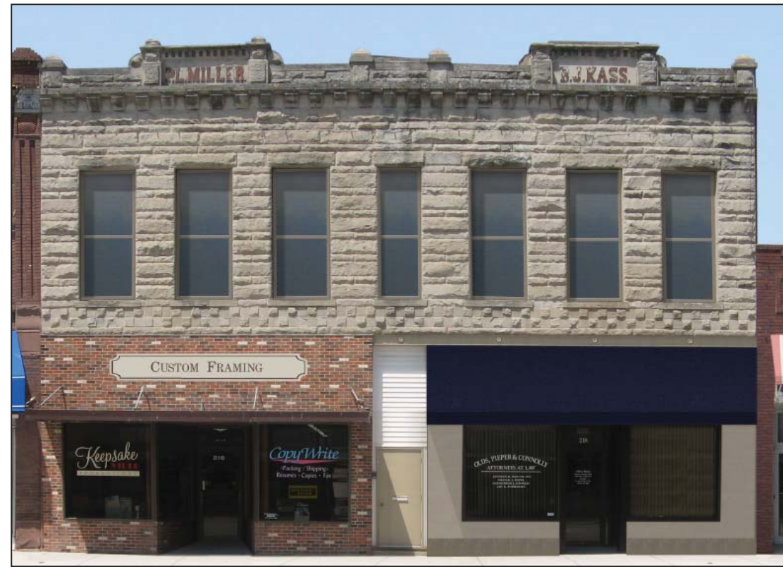
Image 9. Option 3. Otherwise similar to Option 1, stucco is applied only to the lower portion of the north half of the building. The awning is Sunbrella fabric "Navy" (#4626). The signboard shape is different. The font used on the signboard is Times New Roman.
