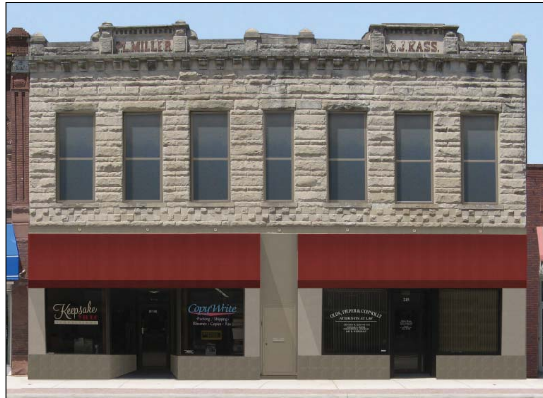
Image 19. Option 10. Otherwise similar to Option 6, the porcelain tile is applied to the entire sidewalk-level bulkhead. The porcelain tile is similar to American Olean "Sand Swept". Both awnings are Sunbrella fabric "Terra Cotta" (#4622).
