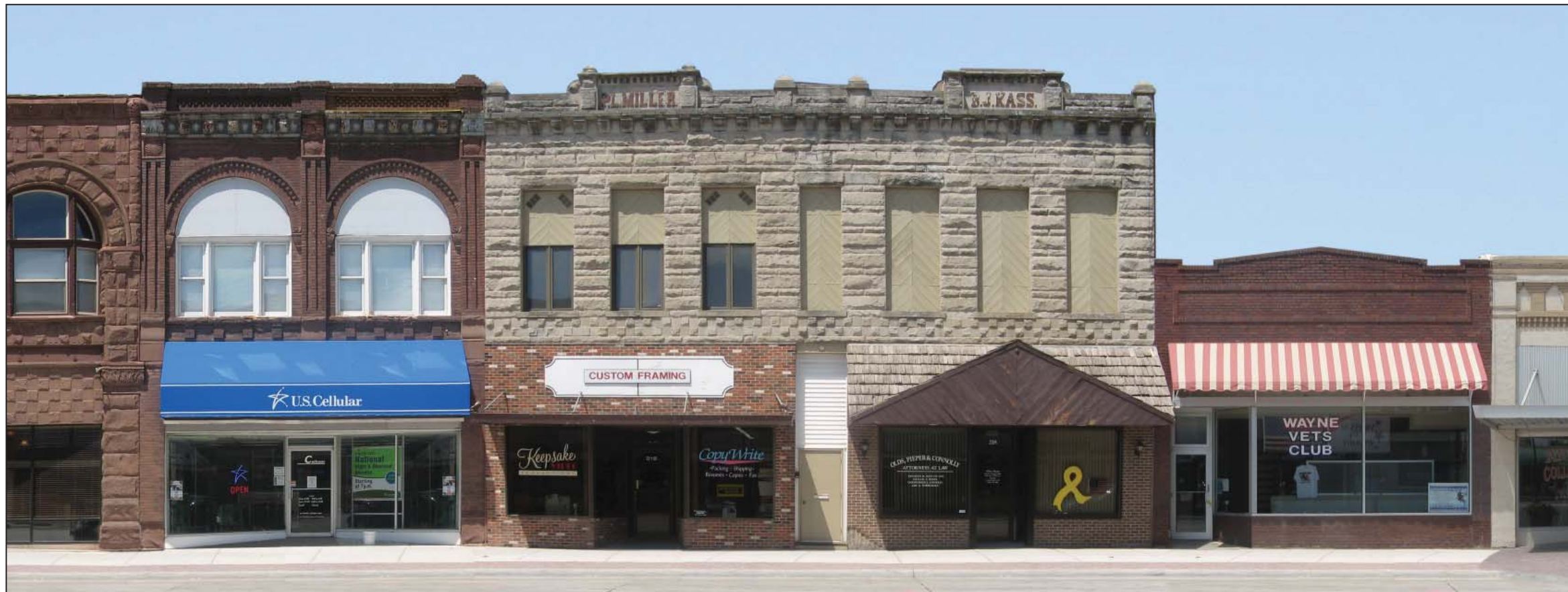
Image 1. Existing Condition. The Miller-Kassler Building is located on the west side of the 200 block of Main Street between buildings occupied by U.S. Cellular and Wayne Vets Club. The south half of the building is occupied by Custom Framing. The north half of the building is occupied by Olds, Pieper & Connolly, Attorneys.
