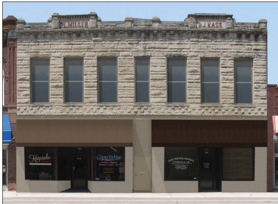
Image 18. Option 9. Otherwise similar to Option 6, stucco is applied to the entire lower portion of the facade. Porcelain tile is not used. The south (left) awning is Sunbrella fabric "Cocoa" (#4676). The north (right) awning is Sunbrella fabric "Walnut Brown Tweed" (#4618).
