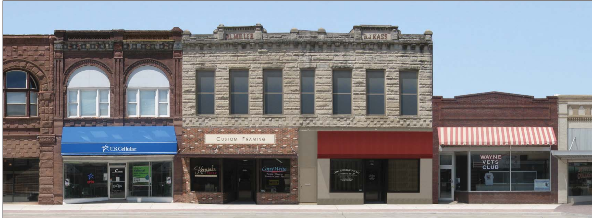
Image 4. Option 1. The stucco used on the lower portion of the north half of the Miller-Kassler Building facade is similar in color to the stone that exists on the upper portion of the building. Darker stucco is used above and at the sides of the door in the middle of the building. The central door is painted to match the stucco that surrounds it. The new awning is Sunbrella fabric "Terra Cotta" (#4622). The single course of 12"x12" porcelain tile installed at the base of the north half of the building is similar to American Olean "Broadway Brown". Full-size double hung windows are installed in all second story window openings. The support beam is revealed. The new signboard on the south half of the building is similar in color to Pratt & Lambert "Flax" paint color (#2048). The font used on the signboard is Avant Guard.
