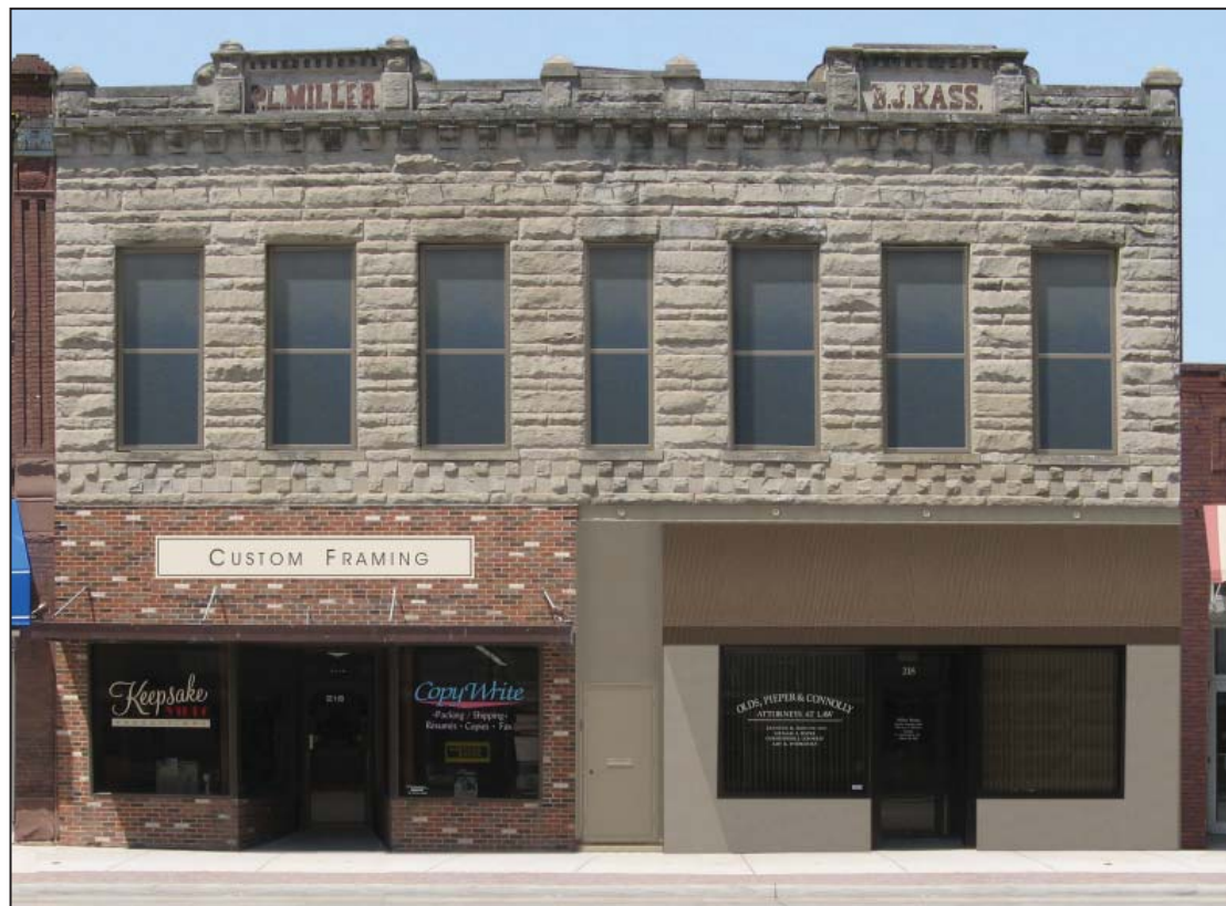
Image 10. Option 4. Otherwise similar to Option 1, stucco is applied to the entire midsection and lower portion of the north half of the facade. Porcelain tile is not used. The awning is Sunbrella fabric "Cocoa" (#4676). The font used on the signboard is Avant Guard.
