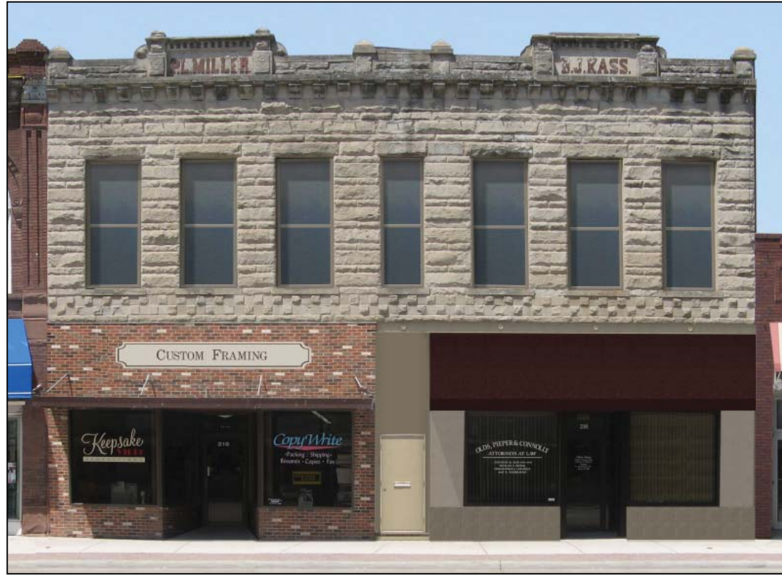
Image 11. Option 5. Otherwise similar to Option 1, porcelain tile is applied to the bulkhead of the north half of the facade. The porcelain tile is similar to American Olean "Sand Swept". The awning is Sunbrella fabric "True Brown" (#4621). The font used on the signboard is Times New Roman.
