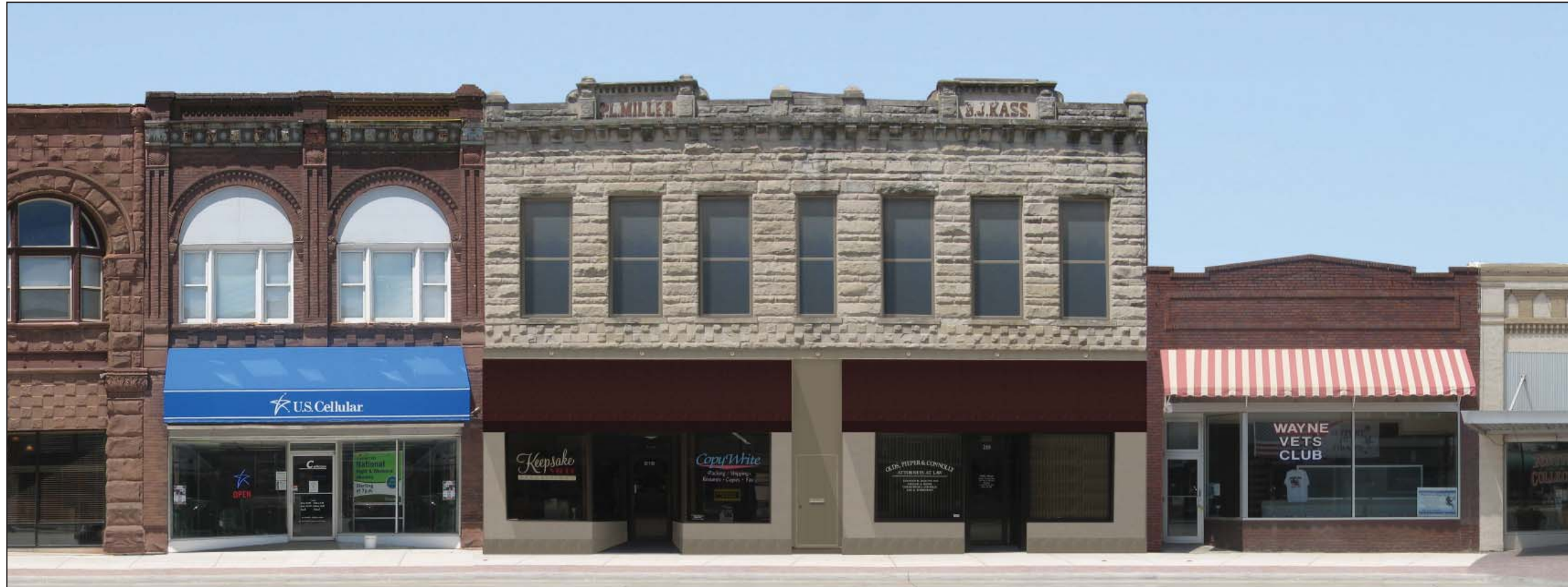
Image 12. Option 6. Stucco used on the entire lower portion of the Miller-Kassler Building is similar in color to the stone that exists on the upper portion of the building. Darker stucco is used above and at the sides of the door in the middle of the building. The central door is painted to match the stucco that surrounds it. The new awnings are Sunbrella fabric "True Brown" (#4621). The single course of 12"x 12" porcelain tile installed at the base of the building facade is similar to American Olean "Broadway Brown". Full-size double hung windows are installed in all second story window openings. The support beam is revealed along the top edges of the awnings.
