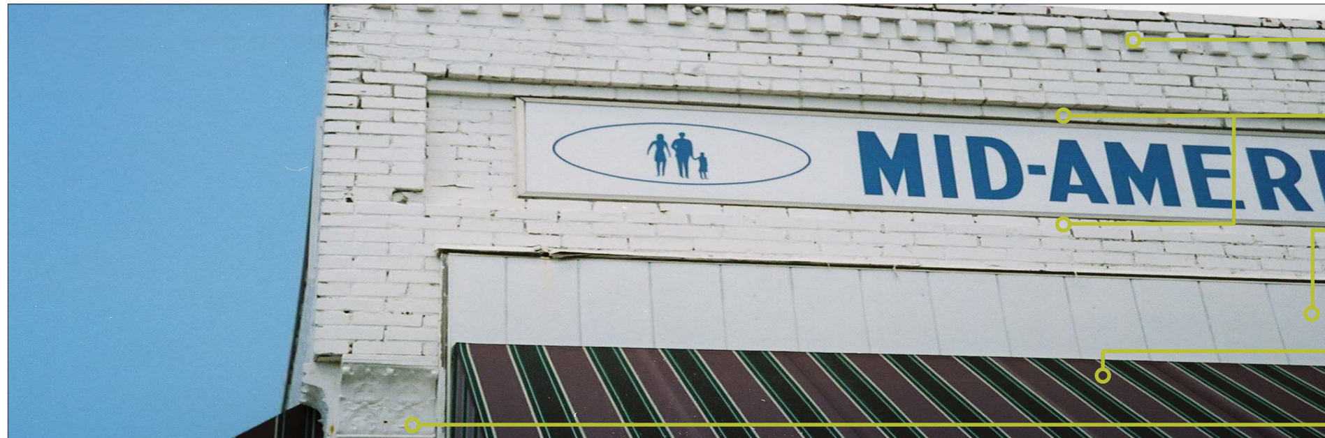
Image 4. Existing Condition (South Façade Detail): Brick dentils accentuate the cornice. The Mid-America sign is set into an elongated rectangular recess in the brickwork. The bulkhead appears to overlap some of the building face brick, which likely exists above the corner column capital, similar to the condition above the storefront window on the west wall. The awning is mounted on the bulkhead. The uneven surface of the bulkhead cladding, as well as the lack of flashing along the top edge of the awning, results in rainwater leakage along the top edge of the awning.
