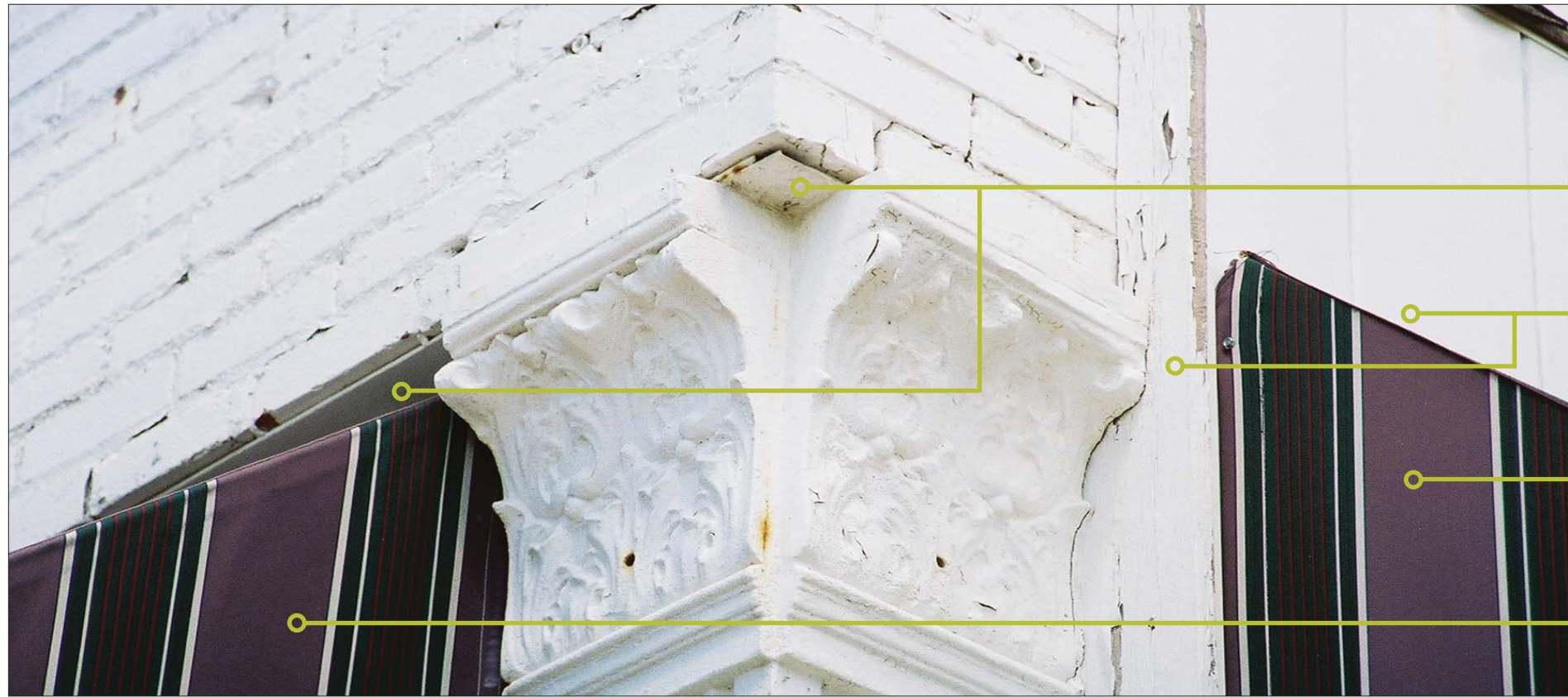
Image 3. Existing Condition (Southwest Corner Detail): The building's original corner cast iron column, with a classical decorative capital and other intricate detailing, remains exposed. This corner column and the other cast iron columns on the façade are important historic elements of the building, all worthy and deserving of preservation and enhancement. This image illustrates two existing awning-mounting conditions on the building: (1) The west awning is mounted underneath the steel flange that supports face brick above. (2) The south awnings are mounted on the surface of a bulkhead that is built out from the original face brick of the façade. Condition #1 is preferable, since it reveals, respects, and visually reinforces the inherent structure of the original building façade. Placement of the top edge of the awning beneath the steel flange also has the advantage of protecting against rainwater leakage at that location. Removal of the built-out bulkhead above the south storefront windows would, presumably, reveal the full height of all the original cast iron columns on the south façade.
