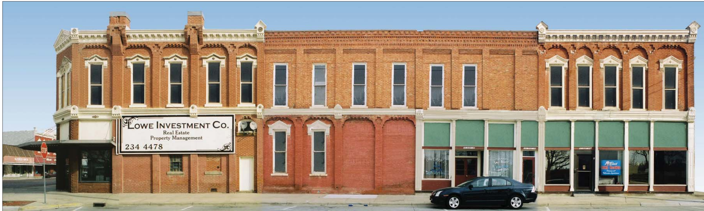
Image 5. Proposed East Railroad Street Façade Improvements. The changes proposed for this façade of the Lowe Building include restoration of the full-height double hung windows and installation of full-height storm windows on the second floor. Removal of the solar collector in one of the second story windows (see Image 4) and restoration of the original window is recommended. This view also shows all of the transom panels in the first floor storefronts painted uniformly.
