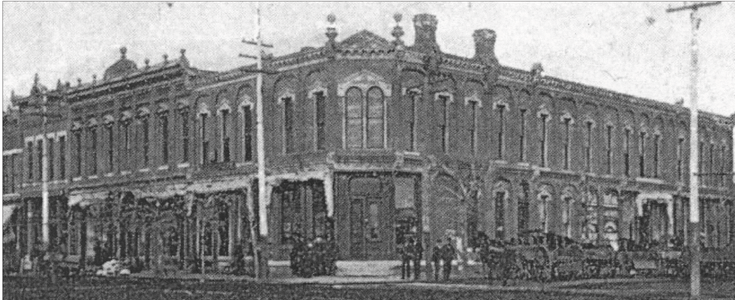
Image 1. Historic Photograph. The two-story Lowe Building, located on the northeast corner of the intersection of Central Avenue and East Railroad Street, is pictured in the late 1800s or early 1900s. The building has cast iron storefronts, a pressed-metal cornice, and pedimented window hoods.
