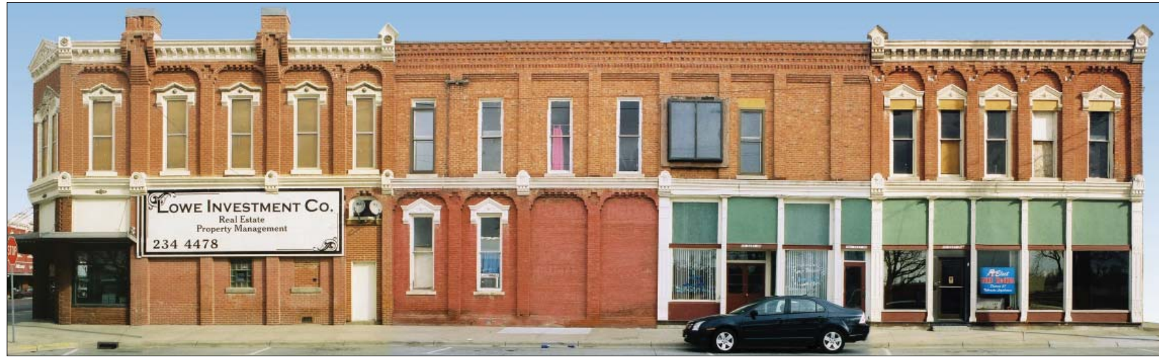
Image 4. Existing Building. The East Railroad Street façade of the portion of the Lowe Building studied for this project (the portion to the right of the “Lowe Investment Co.” sign in this photograph) was altered at some point in the early twentieth century. The midsection of this façade, where the pressed metal cornice no longer exists, was partially replaced in the early 1900s, probably due to structural failure or deterioration of the face brick. The simplified brick cornice and plain second-story window openings on the replacement façade reflect the general move away from ornamented façades in commercial building design in the twentieth century.
