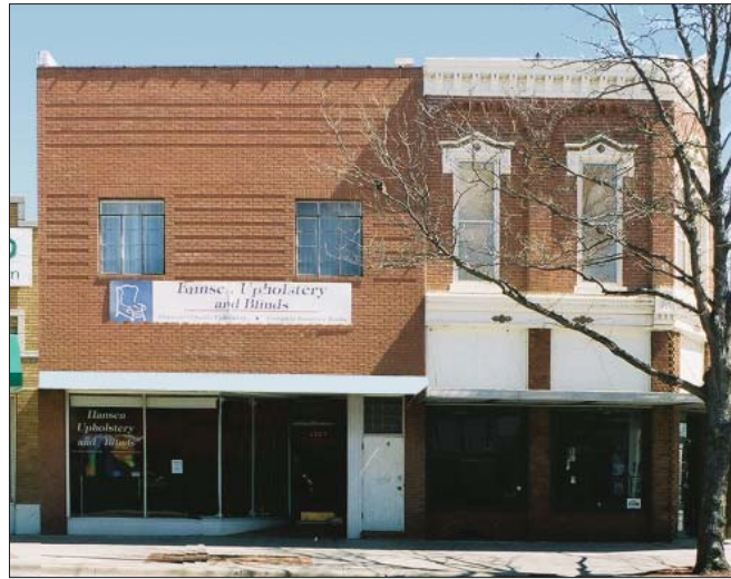
Image 3. Existing Building. The Central Avenue façade of the portion of the Lowe Building studied for this project (storefront on the left in this photograph) was replaced in the early-to-mid-twentieth century. The original ornate brick façade of the late 1800s, shown in Image 1, was replaced with a simplified, yet carefully detailed, “modern” brick façade. The three tall second story windows in the original façade were replaced with two shorter, nearly square windows, and the façade brickwork was accentuated with several horizontal reveals, giving the upper façade a visual horizontality that contrasts with the façade of the original portion of the Lowe Building façade remaining to the right in the photograph.
