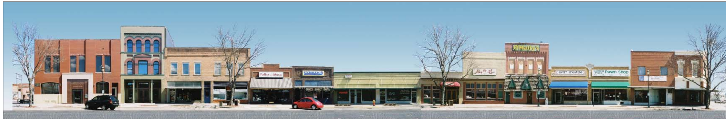
Image 2. Existing Streetscape. The portion of the Lowe Building studied for this project (second storefront from the right) is shown in the context of this block-long row of commercial buildings on the east side of Central Avenue.
