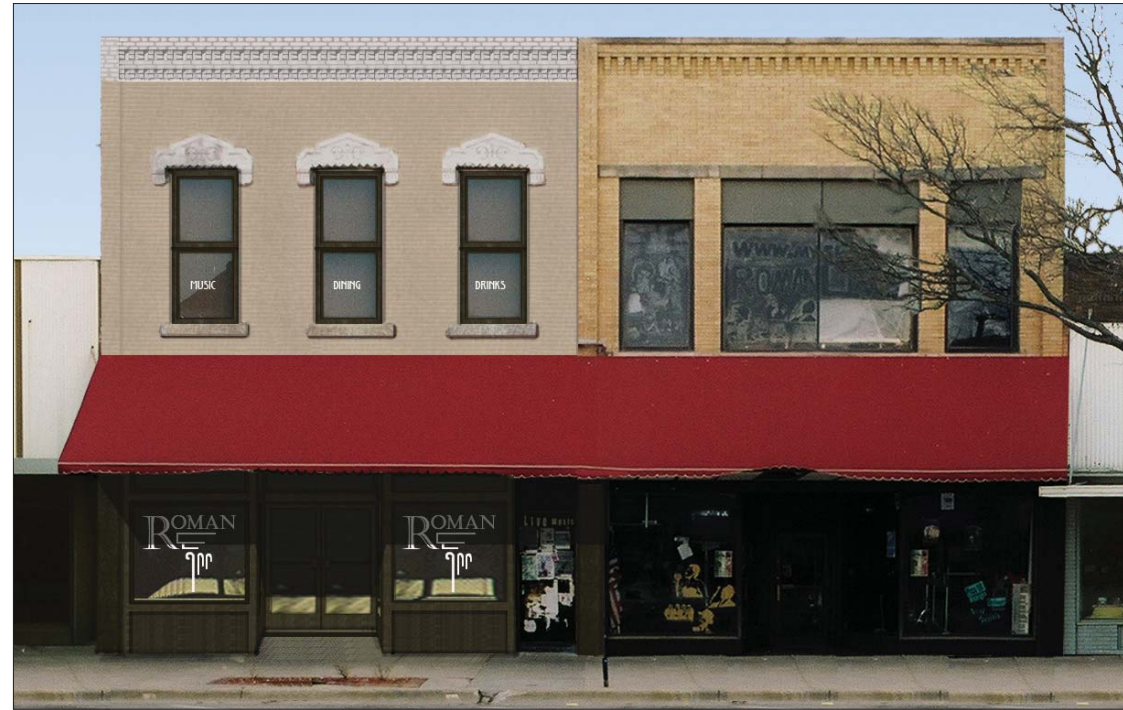
Image 5. Option 1.2: The brick on the second story of the Leach Building is repainted gray, similar to the existing color of the painted brick.
