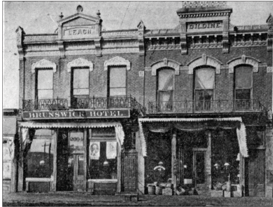
Image 1. Historic Photograph: The image shows the original pair of buildings—the Leach and the Dildine—that today house the Roman nightclub on the first floor.
