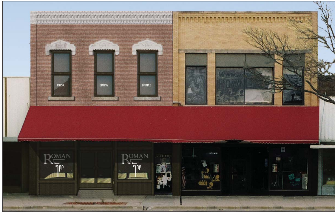
Image 4. Option 1.1: In the Option 1 series, the current storefront of the original Leach Building is replaced with an anodized aluminum (bronze-colored) and glass storefront system that emulates the original historic storefront (see Image 1). Also, the second story windows are replaced with metal bronze-colored double hung windows. Option 1.1 shows removal of paint on the brick of the upper story of the Leach Building. The decorative brickwork on the cornice is painted white to match the window hoods. A new graphic logo (see Image 11) is applied to the storefront windows.
