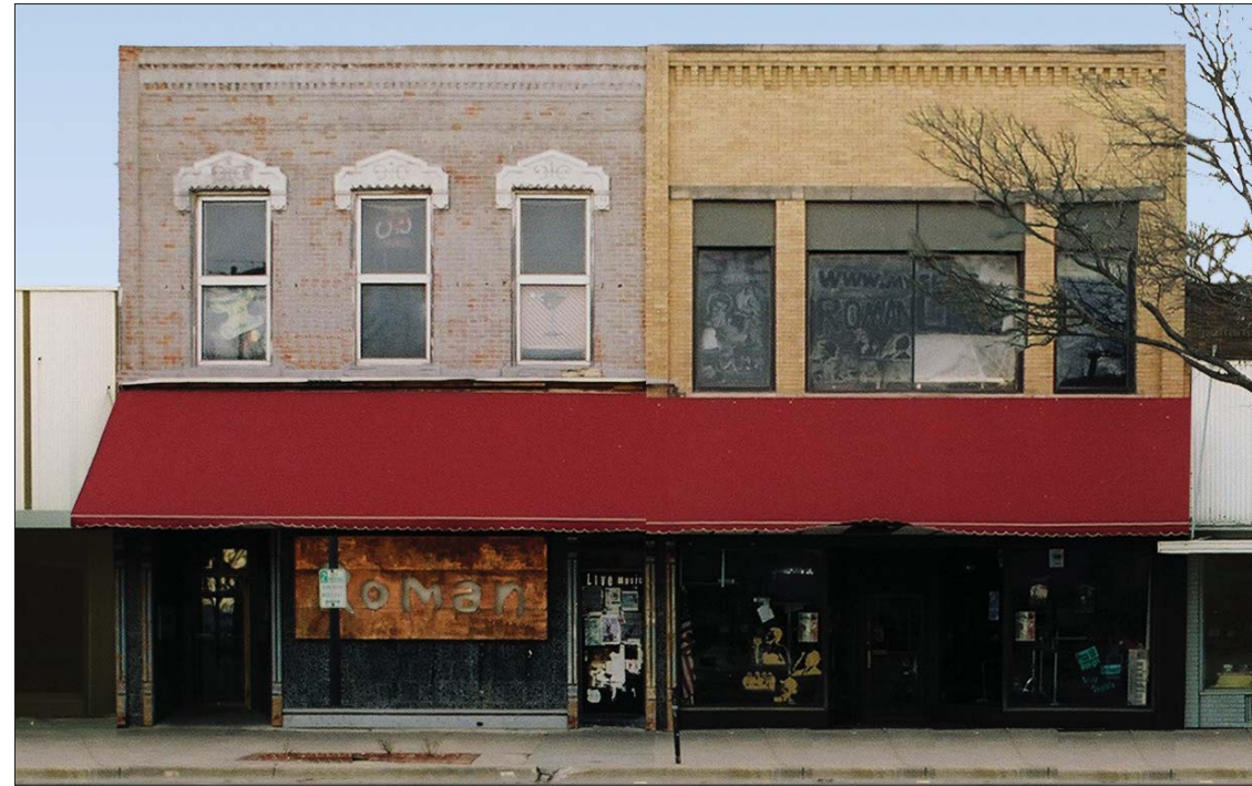
Image 2. Existing Condition: The original Dildine Building subsequently was replaced with a new two-story building. The cornice of the Leach Building was removed, and the brick façade was painted. The original window hoods remain. The original first floor storefronts were altered significantly. An awning spanning across the two storefronts was installed recently.
