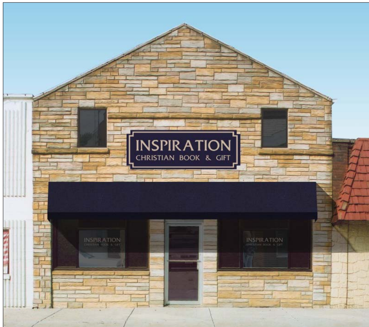
Image 4. Option 1 (East Facade): The awning has closed sides and a 9" valance. The awning projection is similar to that of the adjacent building's roof and aligns with the edge of this roof. The awning fabric is shown in Image 7. The upper-story windows have been replaced and/or cleaned so that the existing painted images on the Plexiglas are removed. Window frames are added to the upper-story windows. (Images 8 and 9 depict the same awning that is described above.)
