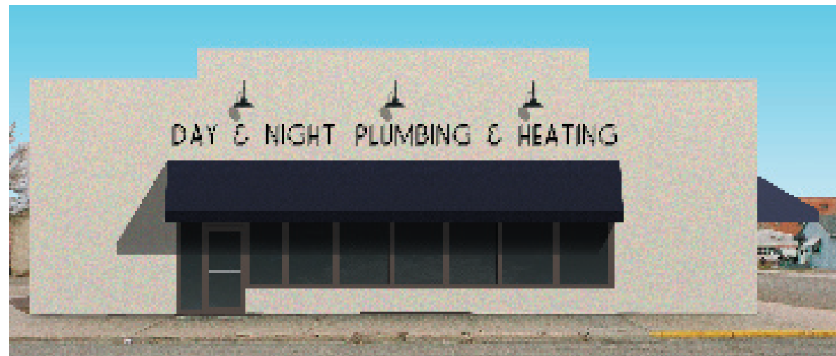
Image 33. Option 3 (South Facade, Alternative Signage): Black, cast metal, Roffe font available from Gemini.
