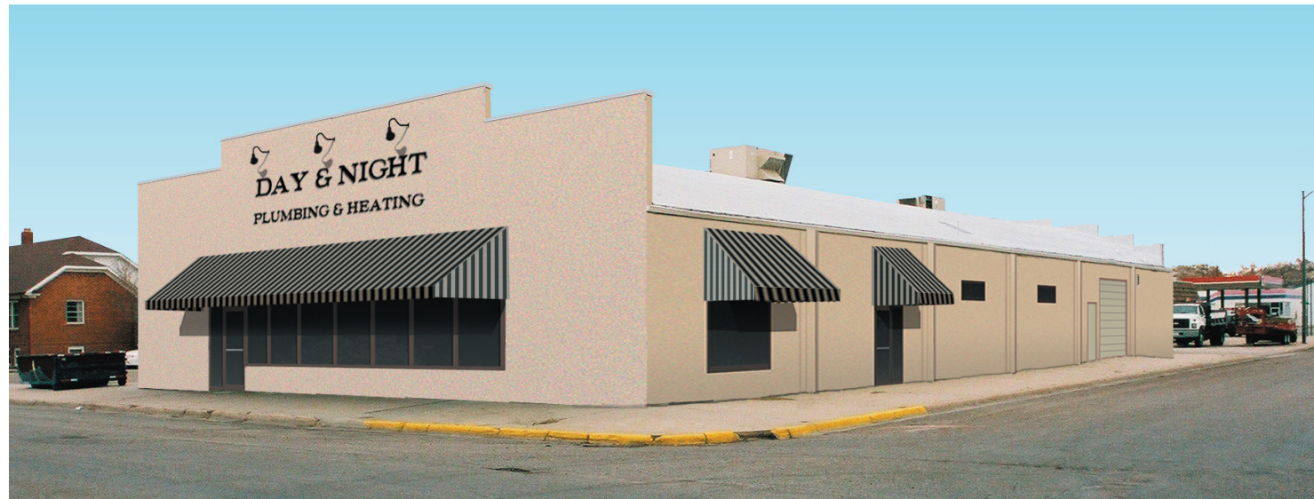
Image 9. Option 2 (Southeast Corner): The stucco or EIFS is similar in color to Pratt & Lambert's "River Sand" paint color (#2265). Smaller scale gooseneck downlighting is used to illuminate the signage.
