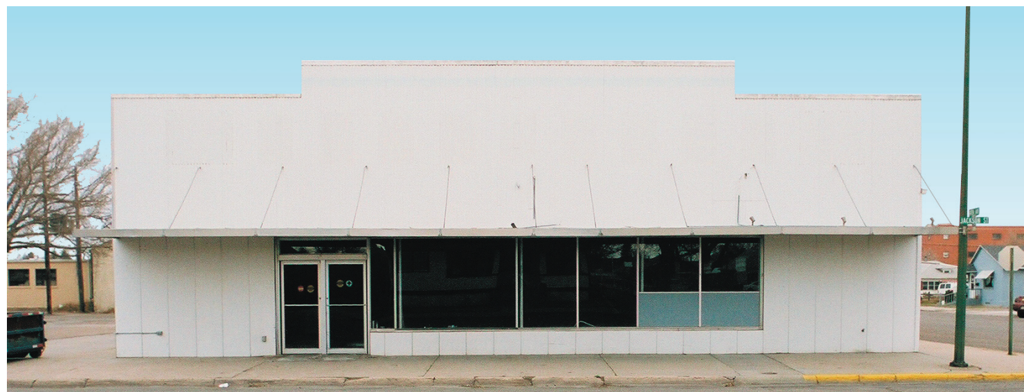
Image 2. Existing Condition (South Facade): The metal canopy and siding are to be removed. Existing windows, frames and mullions will be replaced. The double doors will be replaced with a single door and sidelight.
