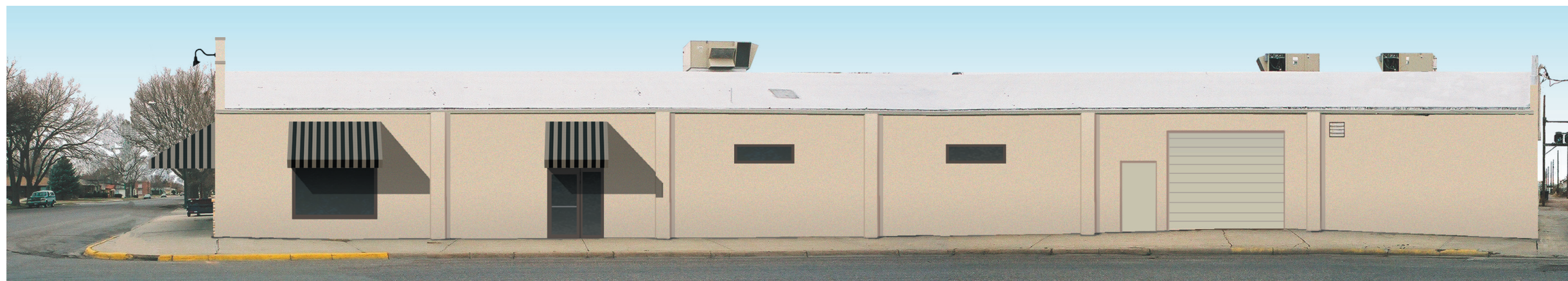
Image 11. Option 2 (East Facade): A new window has been added, as well as a new door with sidelight. A new steel door and overhead door are also shown to the right.
