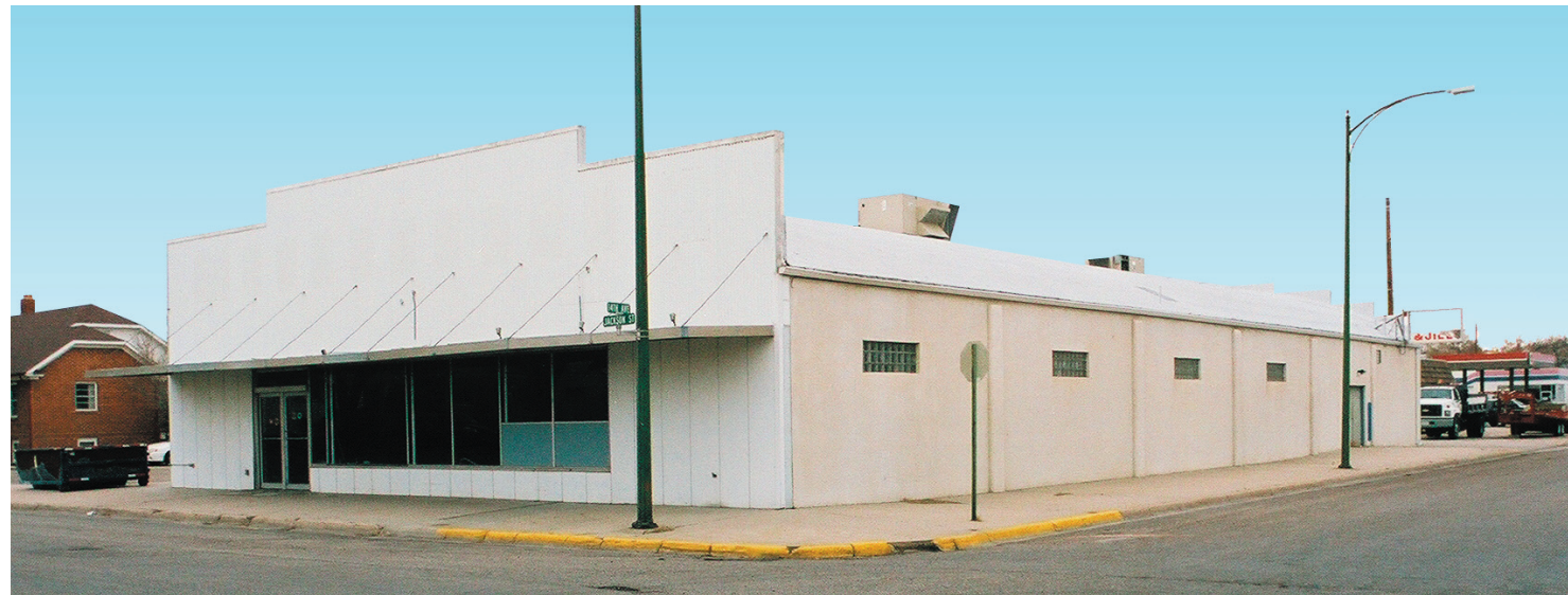
Image 1. Existing Condition (Southeast Corner): Stucco or Exterior Insulation Finish System (EIFS), a synthetic stucco, will be added to the south facade to replace the metal siding to give the building a more cohesive materiality.
