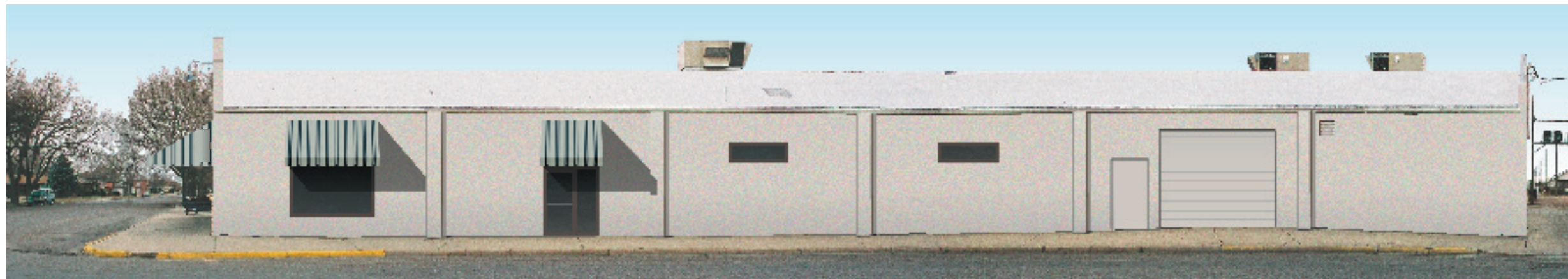
Image 26. Option 5 (East Facade): A new window has been added, as well as a new door with sidelight. A new steel door and overhead door are also shown to the right. The awnings in this option feature a scalloped valance edge.
