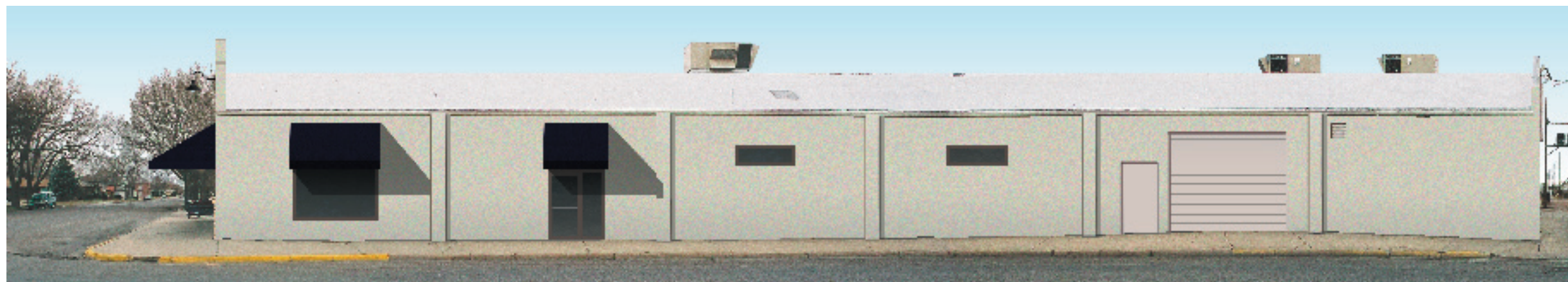
Image 21. Option 4 (East Facade): A new window has been added, as well as a new door with sidelight. A new steel door and overhead door are also shown to the right.
