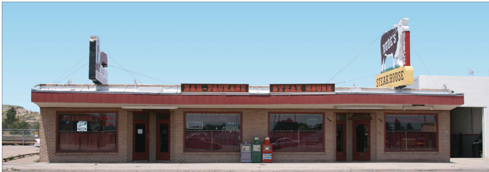
Image 1. Existing Condition (South Facade): The following Options 1, 2, 3 and 4 show the removal of the existing canopy (including the attached signage and lighting), newspaper vending machines, and address numbers. These options also depict a reconfiguration of the entryways in which a pair of recessed, bronze double doors have been installed. The two existing signs on the roof remain in their current location in Options 1, 2 and 3.
