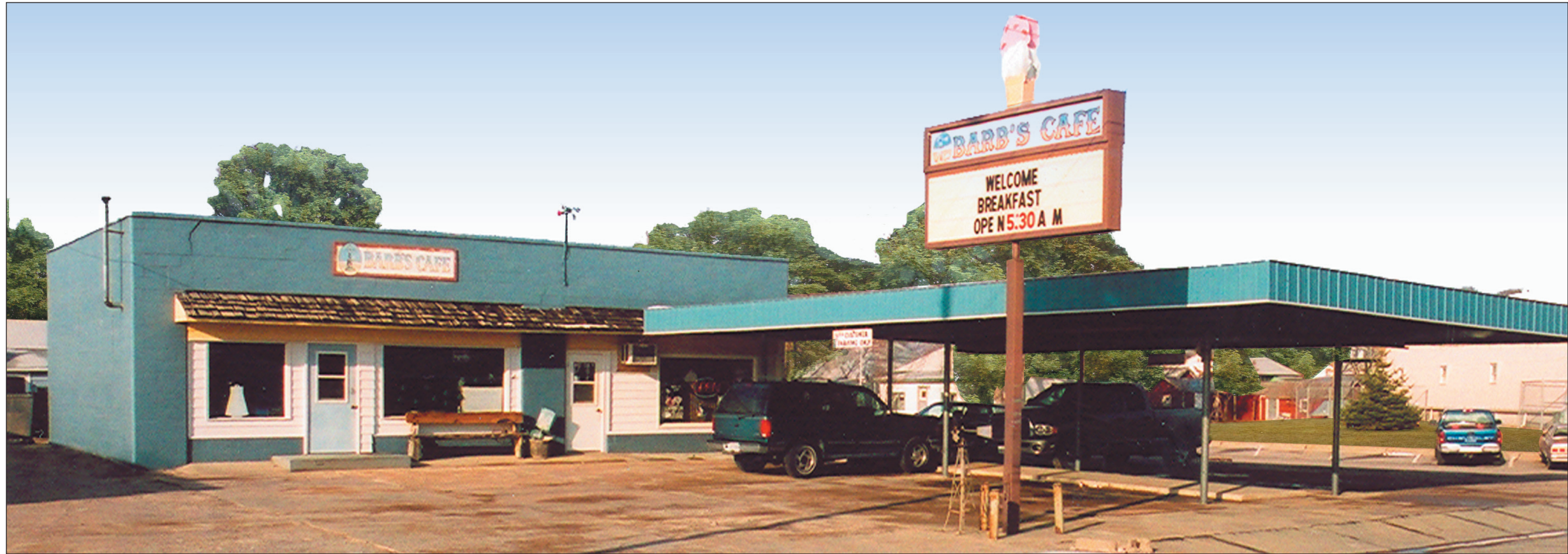
Image 3. Existing condition. Southwest corner.
