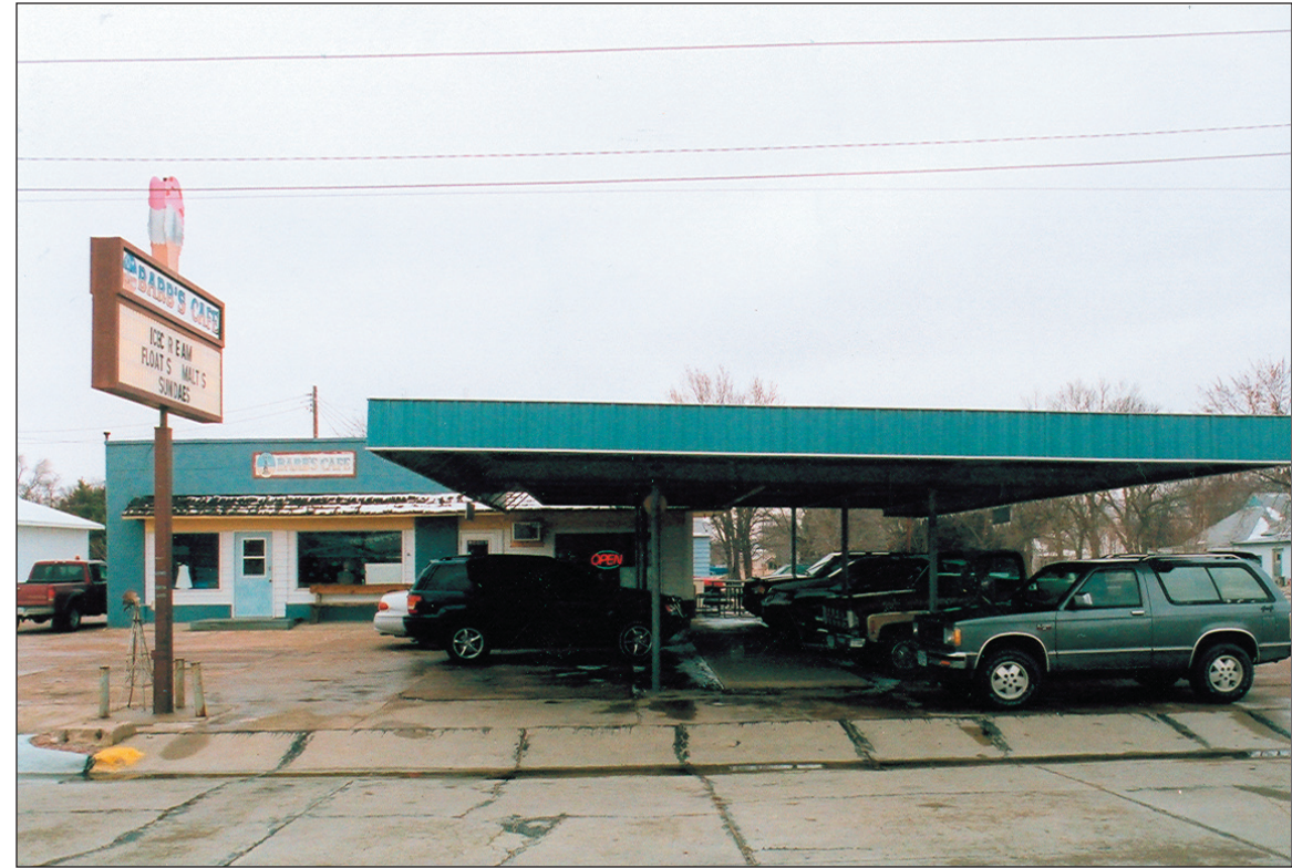
Image 2. Existing condition. South facade.
