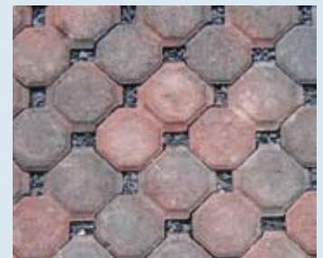
Pervious pavers can reduce impervious surface in developed areas.
