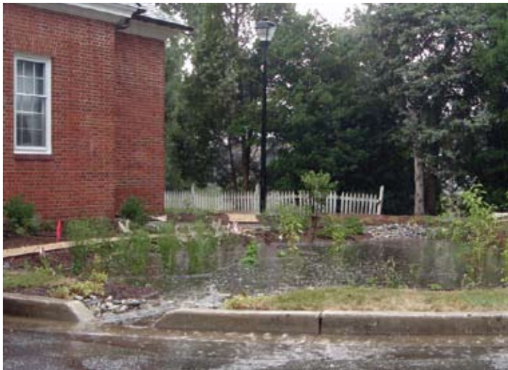
Rain gardens such as this one at the Centreville Library trap runoff and allow it to infiltrate.
