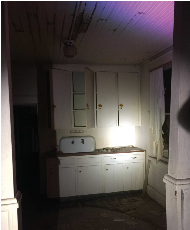
Photo 8: Rear apartment kitchen
