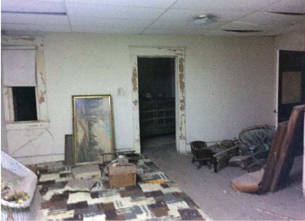
Photo 7: Front room looking west
